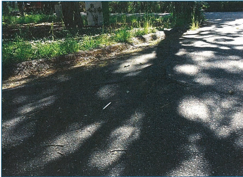
Photo 1 (2017.06.26) – asphalt cracking due to tree root system
