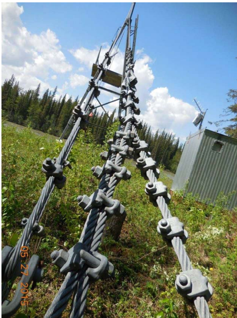
Photograph 5: Finlay River (above Akie River) “home side” clip-type wire rope end connections.
