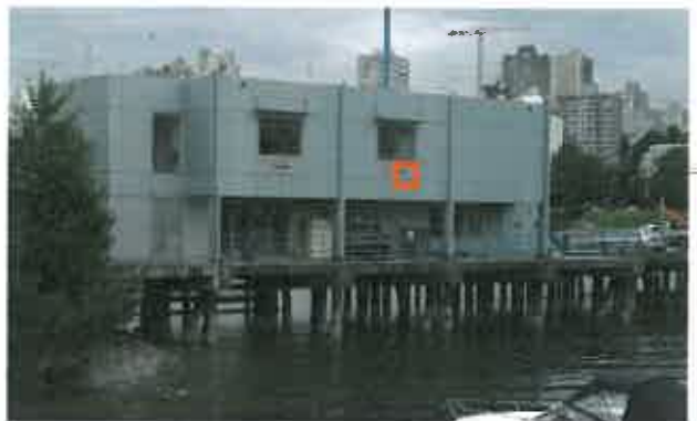
Figure 3 – Exterior condition at location of exploratory opening No. 8.
