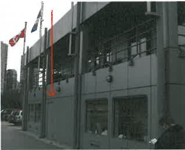
Figure 2.2.2.2 – Several solid swing doors are fully exposed
