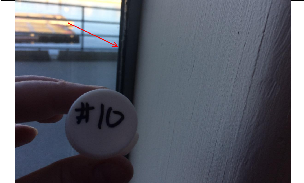
Photo 9 Date: January, 2017 Location: North Window
