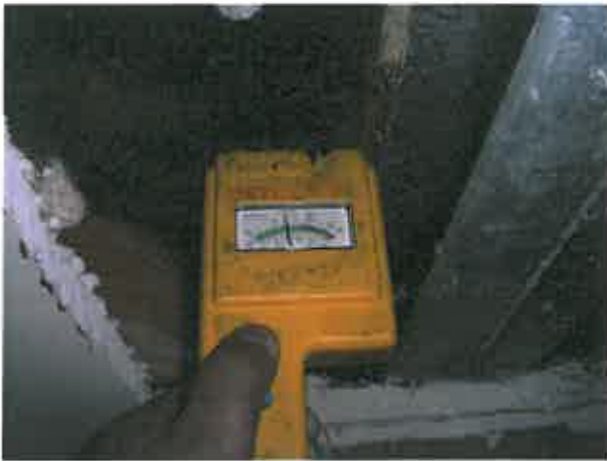
Figure 1.6.1.1: Investigation of a typical exterior wall using a moisture meter.
