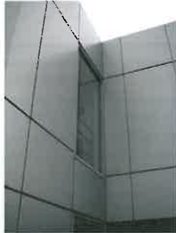
Figure 2.2.1.1 – Storefront glazing locations with no overhang protection
