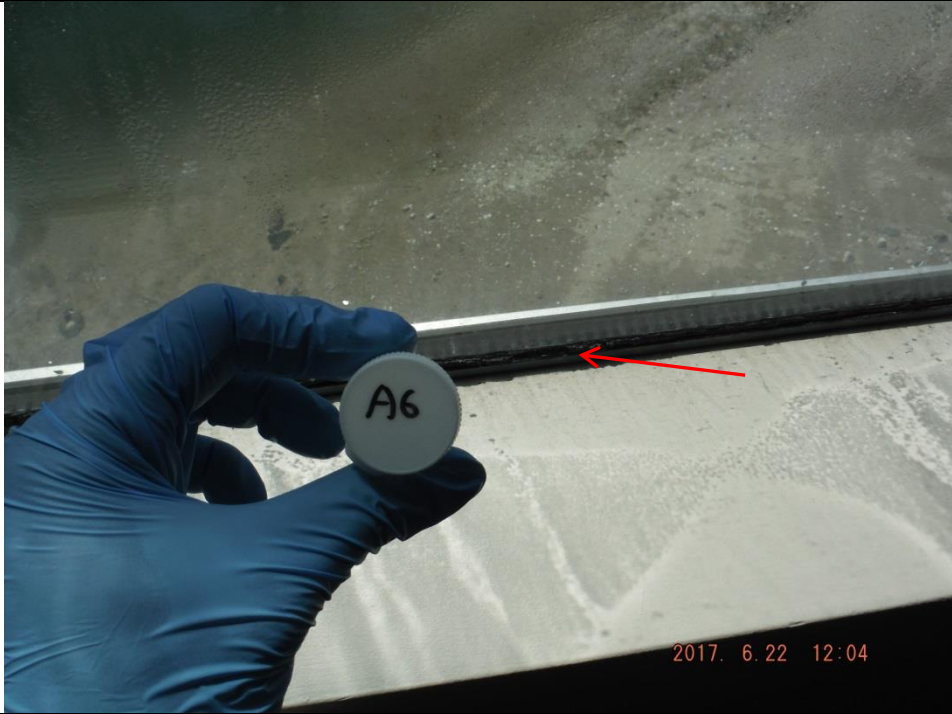
Photo 1 | Date: June 21, 2017 | Location: 2 nd Floor- Cabin 2 Window
