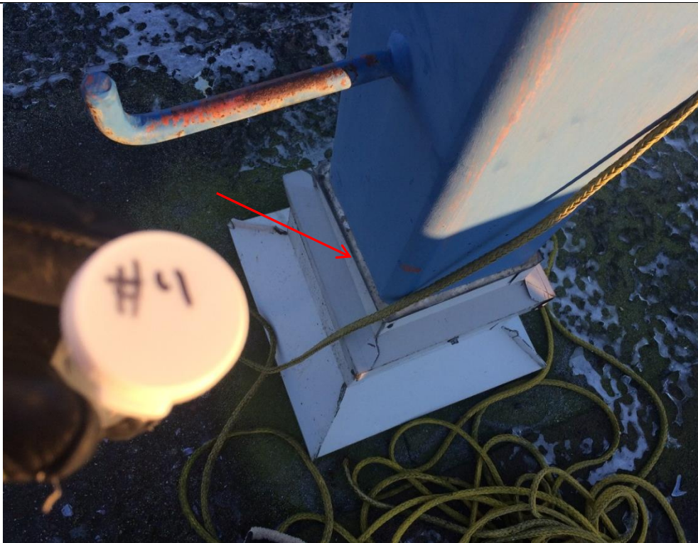
Photo 8 Date: January, 2017 Location: Roof Antenna Pole Description: White Mastic
