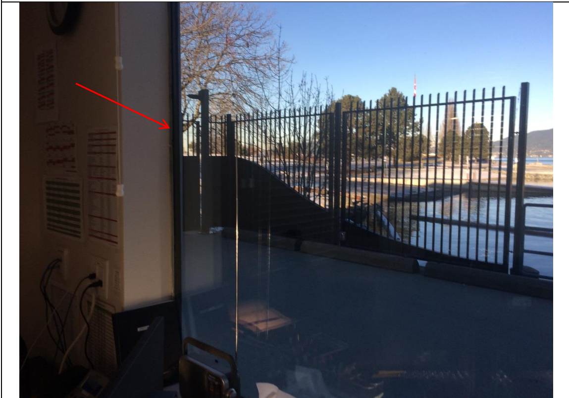
Photo 10 Date: January , 2016 Location: NW Office Window
