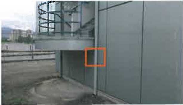
Figure 5 – Exterior condition at location of exploratory opening No. 12.
