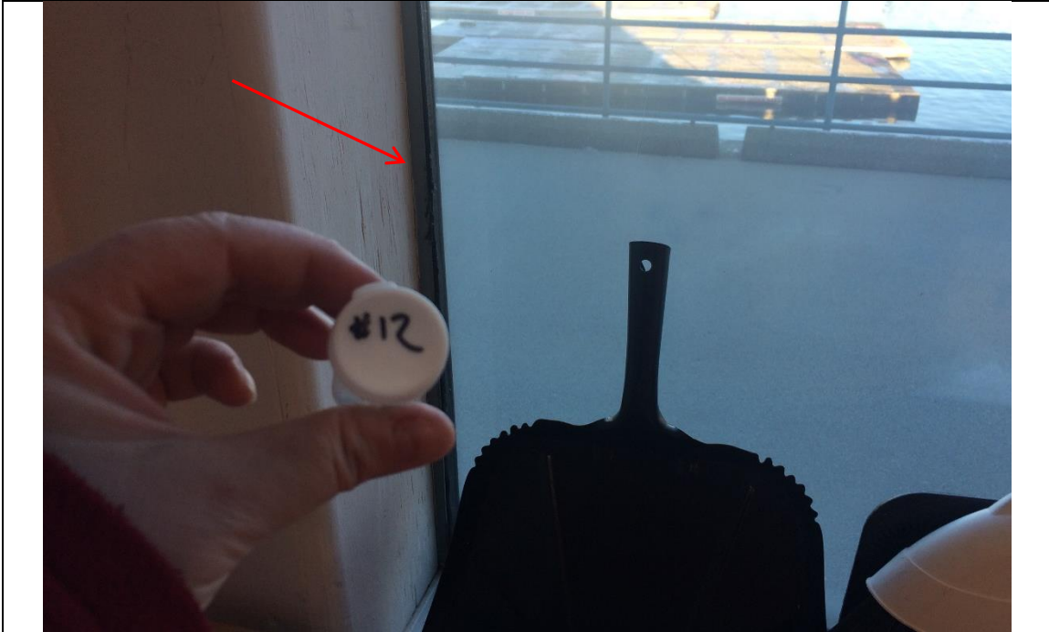
Photo 11 | Date: January , 2016 | Location: NE Window
