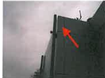
Exterior view of opening area
