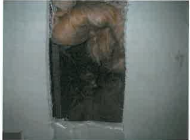
Figure 1.6.2.1: Investigation of exterior wall by means of an interior exploratory opening.
