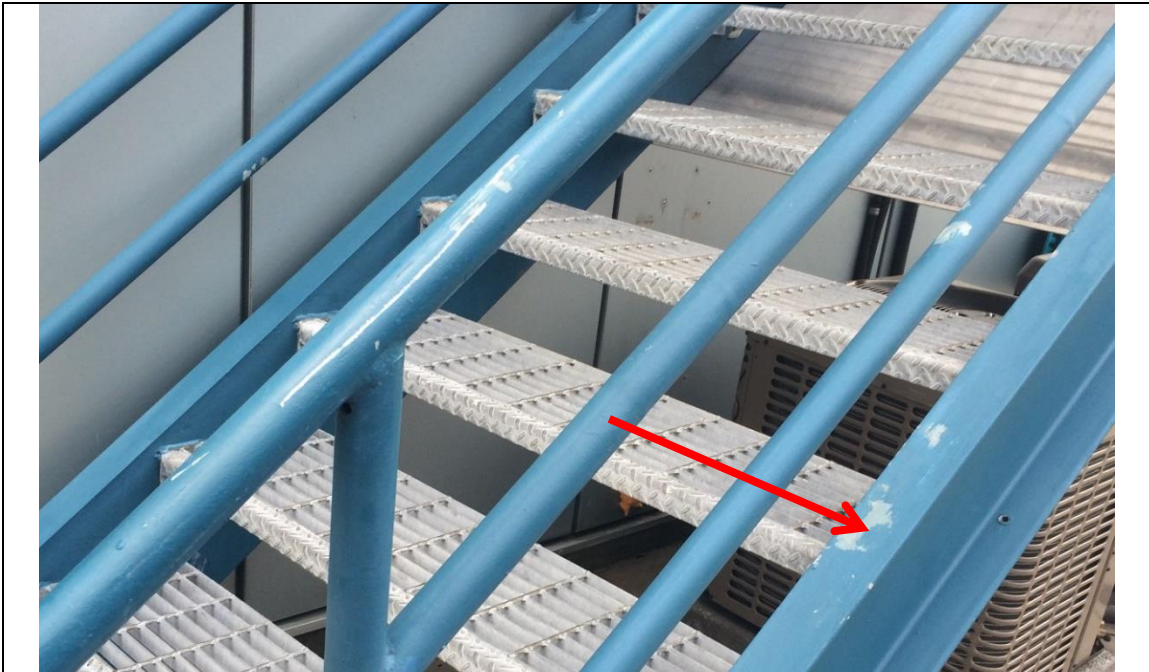
Photo 12 | Date: October 2016 | Location: East Exterior Stair Railing
