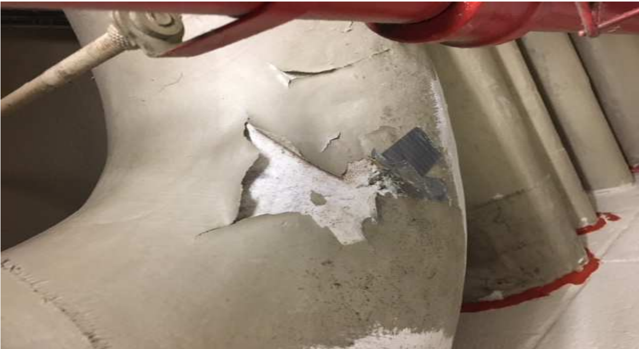
Photo #1. Example of damaged paring cement fitting outside room S-125.
