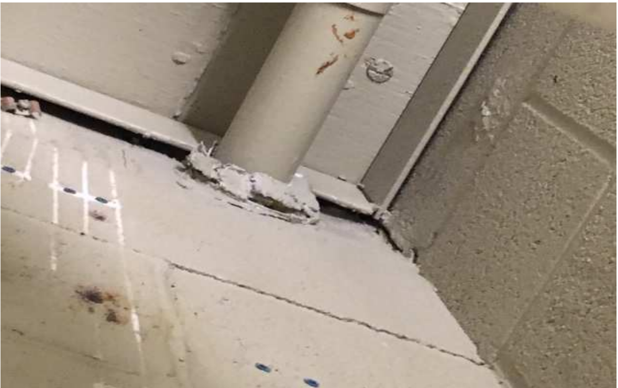
Photo #2. Example of damaged firestop Mechanical Room 331.
