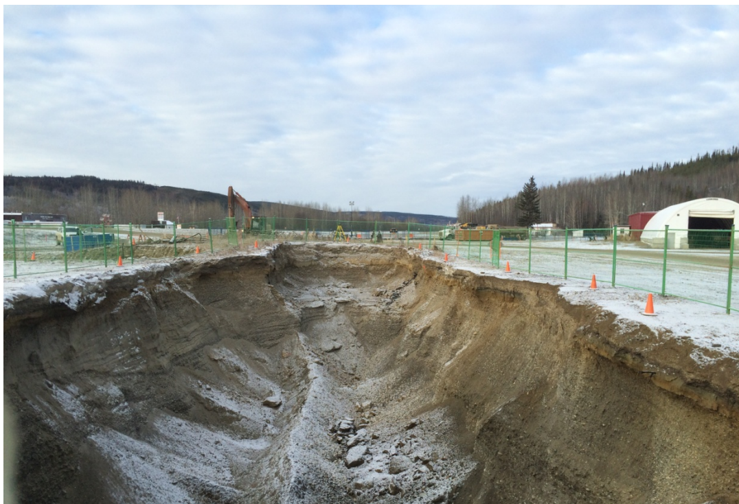
Photograph 6: View of Excavation AEC 3A, looking west on November 16, 2016.
