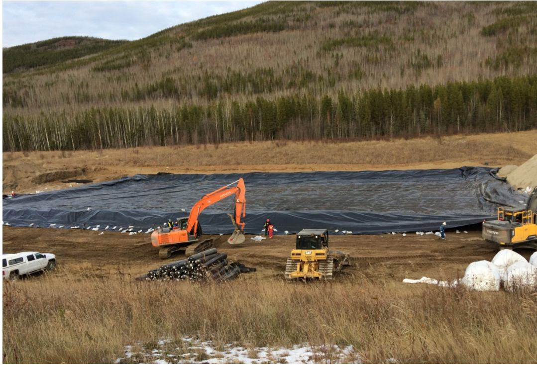
Photograph 3: View of completed Base Liner Installation at STF 1, looking northeast.
