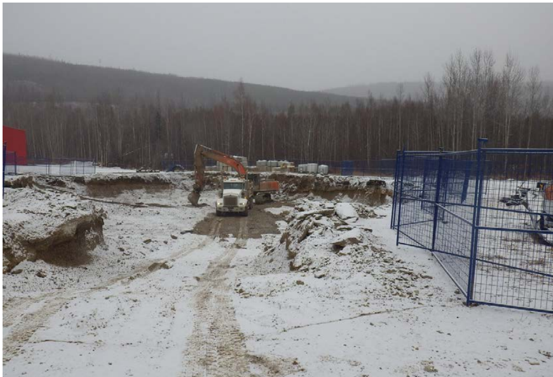
Photograph 8: View of excavation AEC 3C, looking east on November 19, 2016.
