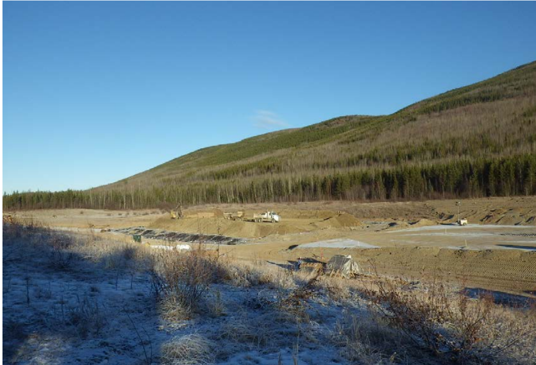
Photograph 1: View of STF construction activities at JJJ Gravel Pit, looking north.
