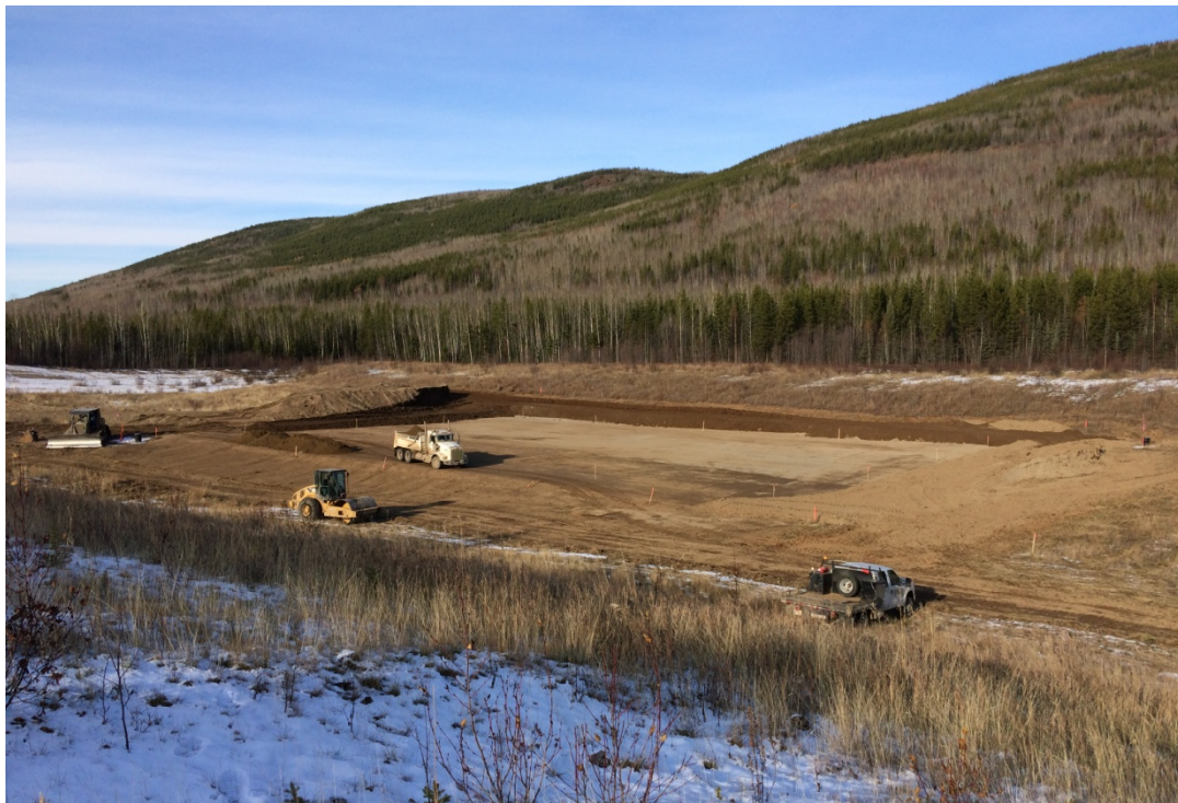
Photograph 2: View of subgrade at STF 3, looking north.
