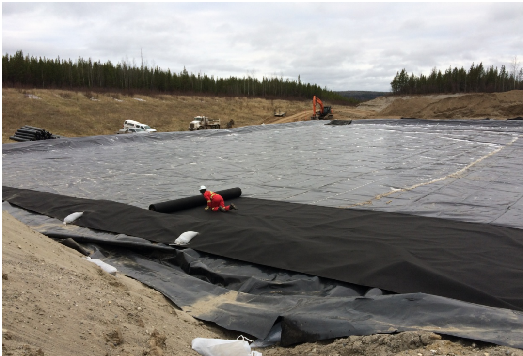
Photograph 4: View of the installation of Geotextile over Base Liner.
