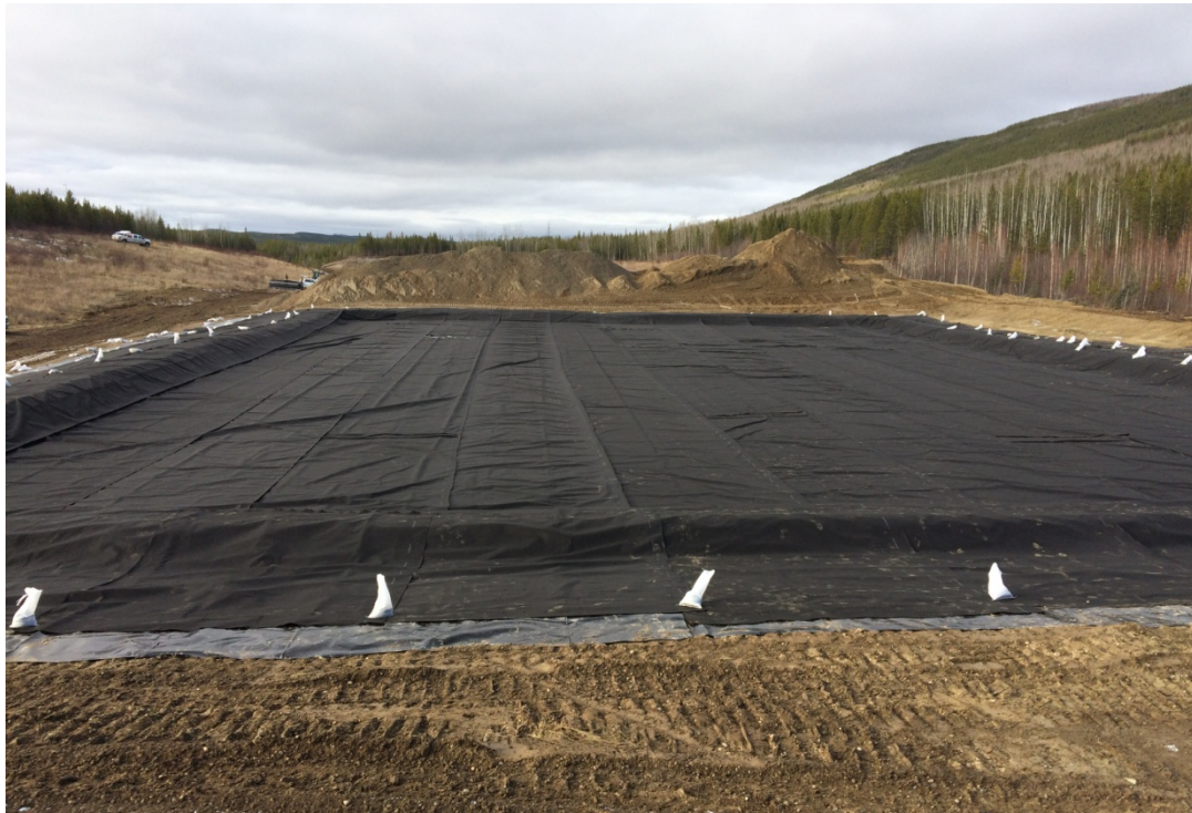
Photograph 5: View of Completed Protective Geotextile installation at STF 1.
