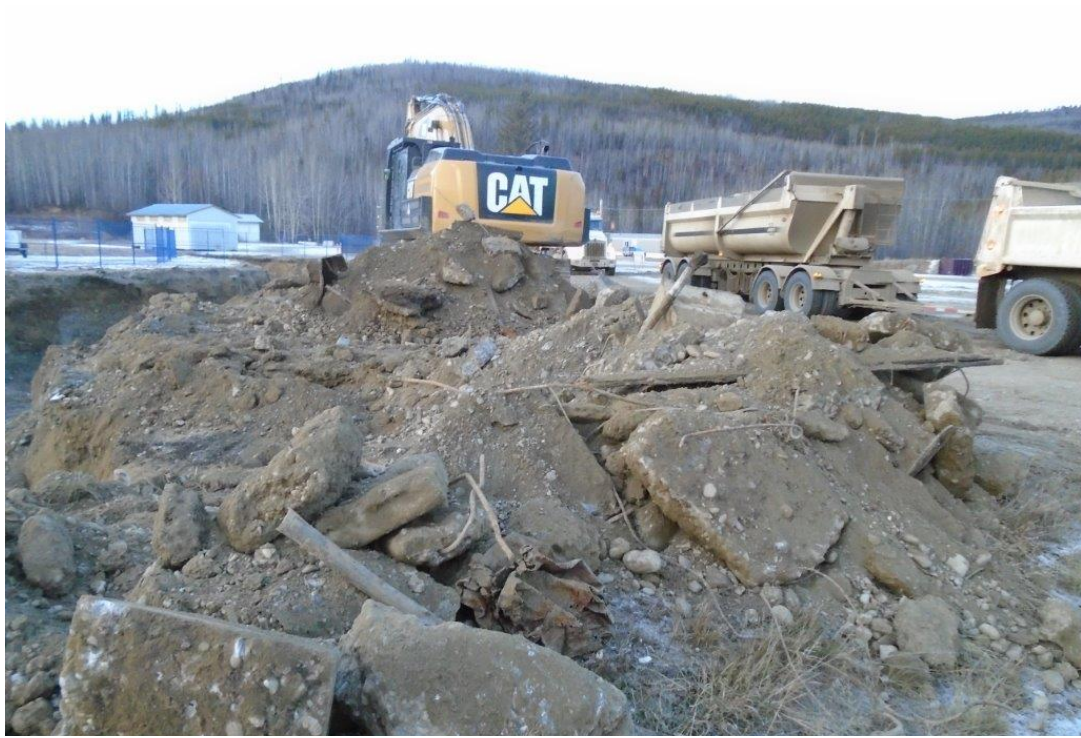
Photograph 11: View of typical debris encountered in shallow soils.
