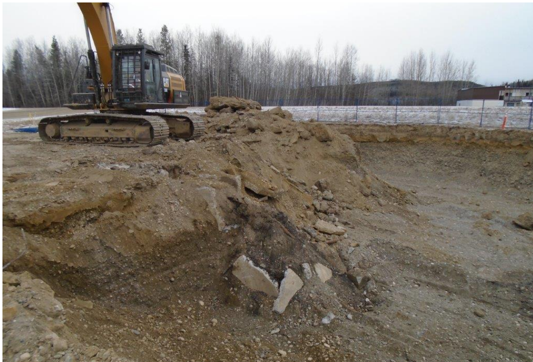
Photograph 10: View of excavation AEC 5.
