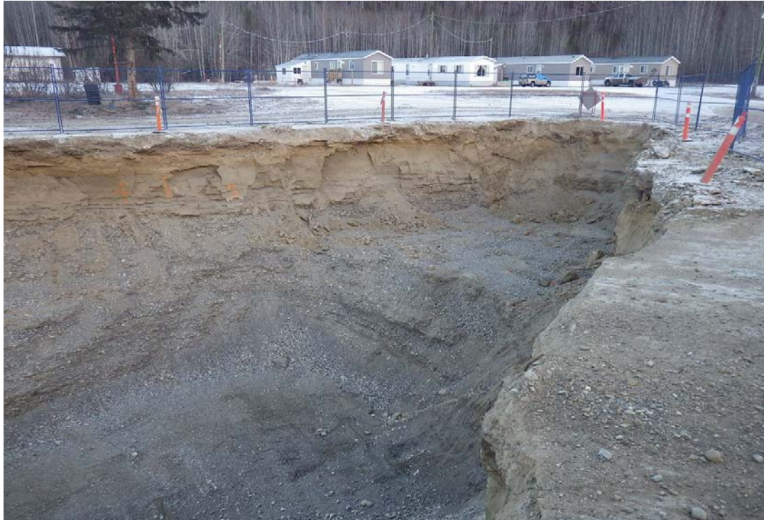
Photograph 7: View of Excavation AEC 1, looking north on November 18, 2016.
