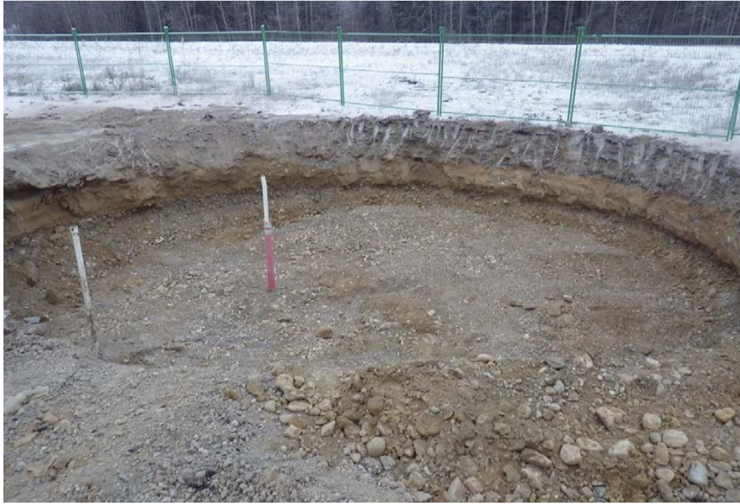
Photograph 9: View of excavation AEC 3D.
