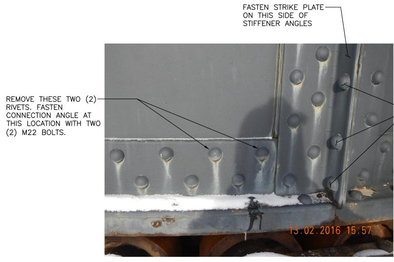
**CONNECTION DETAIL** SCALE: 1:5 300mm 400mm
