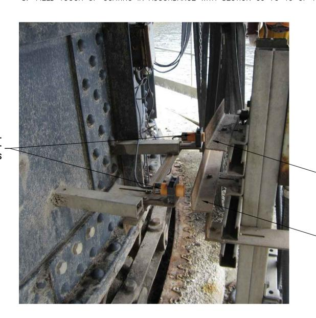
RELOCATE THE FULL OPEN LIMIT SWITCHES TARGETS AND HARDWARE AS NEEDED TO INDICATE THE RELOCATED FULL OPEN LIMIT SWITCHES.
