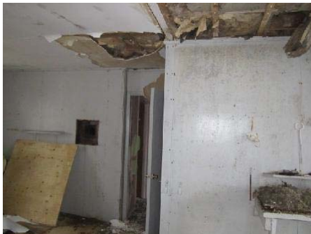
Photo 70: View of collapsed drywall and areas of SVG on drywall in Workshop.
