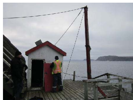
Photo 15: View of lower landing deck, winch house and spar. Note: missing boom.
