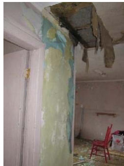
Photo 71: View of collapsed drywall and areas of flaking paint in Hallway 1.
