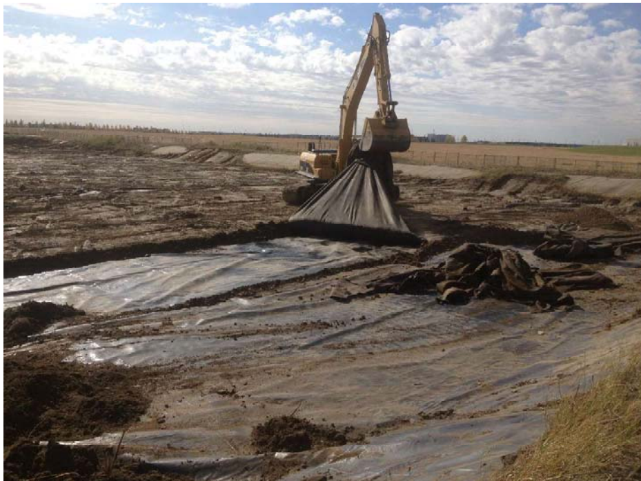
Photograph 9: Removing the top geotextile liner.
