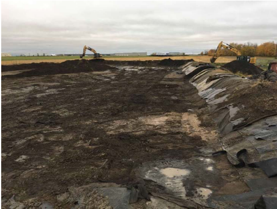
Photograph 11: Removing the liner from the berm and spreading soil in the north cell.
