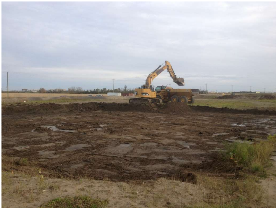
Photograph 6: Removing soil from the north cell.
