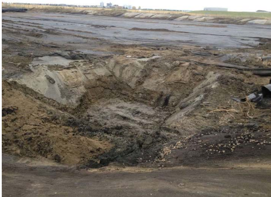
Photograph 8: North sump prior to backfilling.
