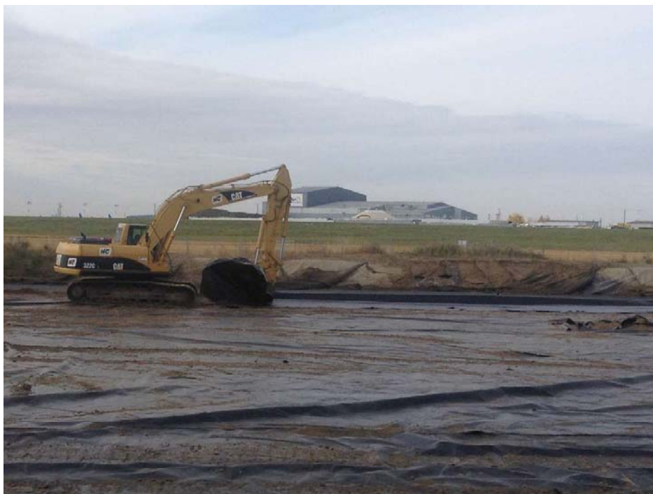
Photograph 10: Removing the second liner.
