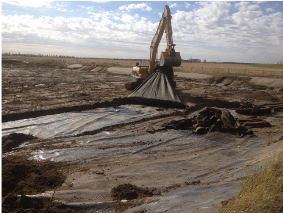
Photograph 9: Removing the top geotextile liner.
