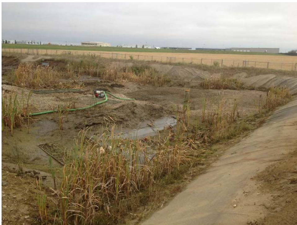
Photograph 4: North sump after pump and treat activities.
