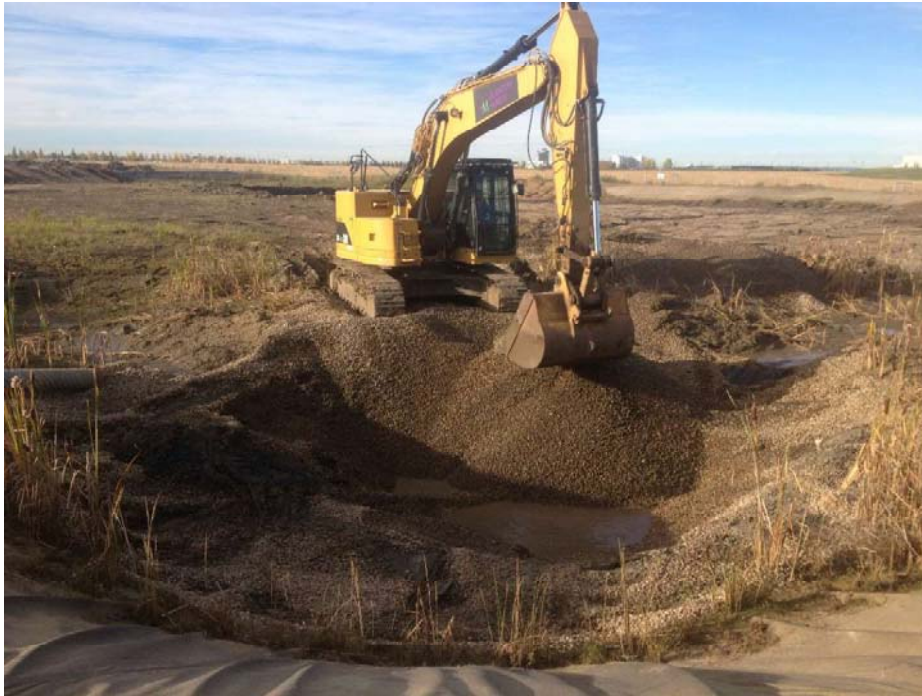
Photograph 7: Removing gravel from the north sump.
