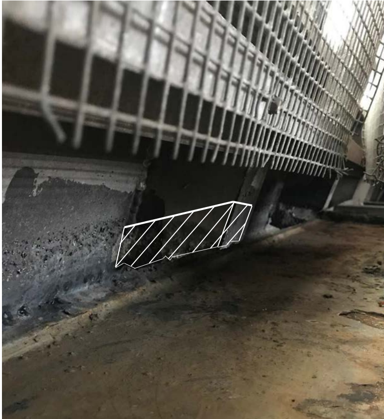
Photograph 1: Funnel side stiffeners to be cropped
