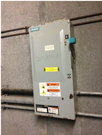
Replace Branch Wiring Devices - 100A Disconnect Switch
