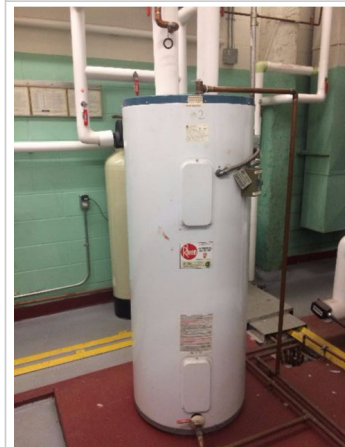
Water Heater - Elec - Comm - 60 Gal
