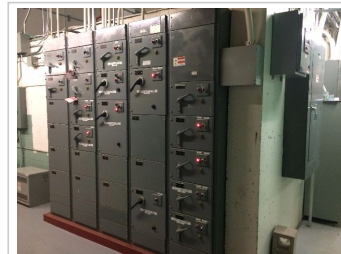
Distribution Equipment - 2000A, 600/347V & 208/120V
