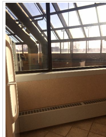
Perimeter Heat System - Hydronic Fin Tube
