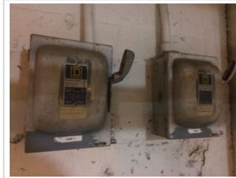
Replace Branch Wiring Devices - 30A Disconnect Switch
