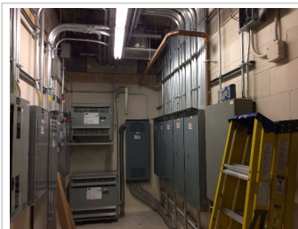
Distribution Equipment - 2000A, 600/347V & 208/120V
