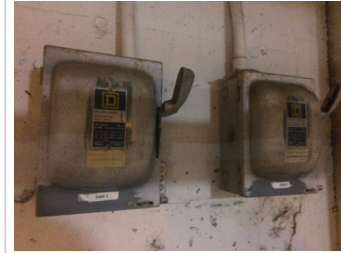
Replace Branch Wiring Devices - 30A Disconnect Switch
