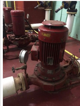
Heating Distribution - Hot Water Piping &amp; Pumps
