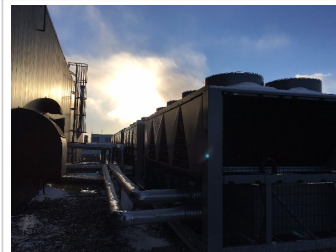
Chiller - Reciprocating - Air-Cooled - Chillers 1-4 & pumps
