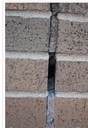
Control Joint Repairs
