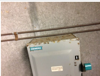
Replace Branch Wiring Devices - 100A Disconnect Switch
