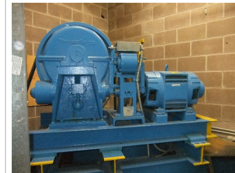
Traction Geared Passenger Elev - Low-Rise - 3
