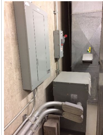
Relocate Transformers in Front of Electrical Components
