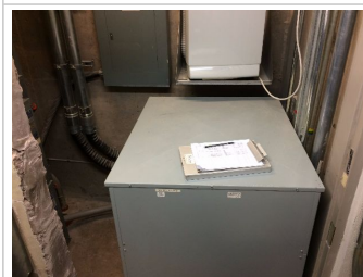
Relocate Transformers in Front of Electrical Components
