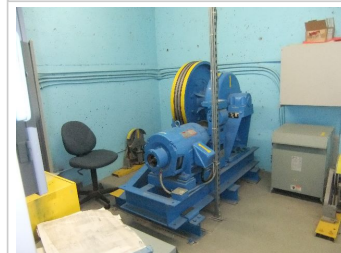
Traction Geared Passenger Elev - Low-Rise - 1,2
