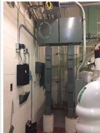
Distribution Equipment - 2000A, 600/347V & 208/120V
