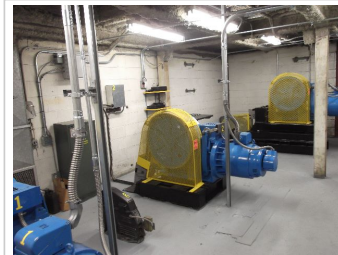
Installation of elevator machine room equipment component guarding.
