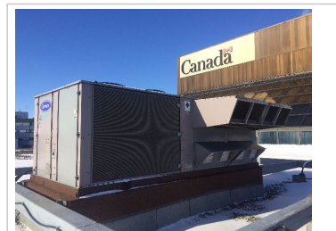
Rooftop Unitary AC - Elec. Heat/Cooling
