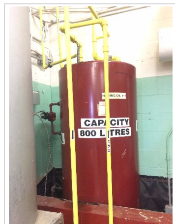
Aboveground Fuel Tank - Steel - 800L
