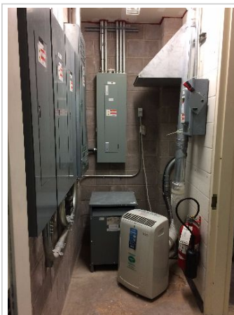
Relocate Transformers in Front of Electrical Components
