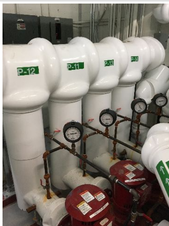
Chiller - Reciprocating - Air-Cooled - Chillers 1-4 & pumps
