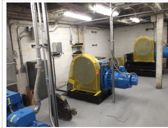
Installation of elevator machine room equipment component guarding
