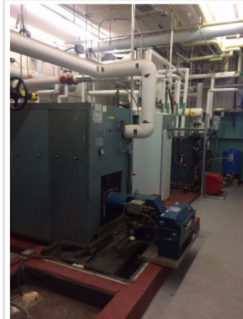
Boiler HW - Gas/Oil-Fired
