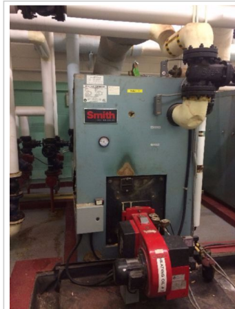
Boiler HW - Gas/Oil-Fired
