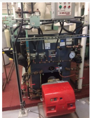
Boiler Steam - Gas/Oil-Fired
