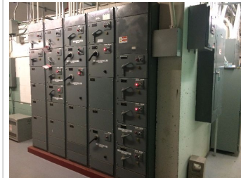
Replace Motor Control Center
