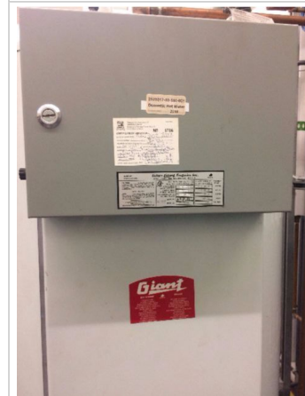
Water Heater - Elec - Comm - 120 Gal - New
