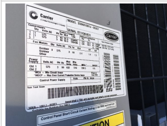
Chiller - Reciprocating - Air-Cooled - Chillers 1-4 & pumps
