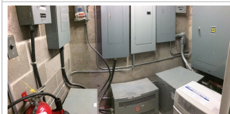
Relocate Transformers in Front of Electrical Components
