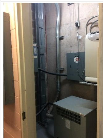
Relocate Transformers in Front of Electrical Components
