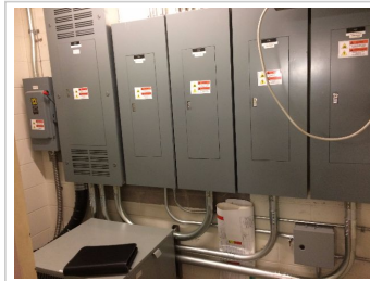
Relocate Transformers in Front of Electrical Components
