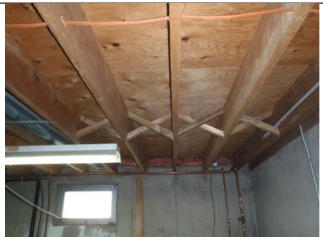
Photo 42 – Main floor joist herring bone bridging
