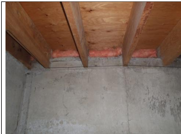
Photo 41 – Main floor joists on basement wall
