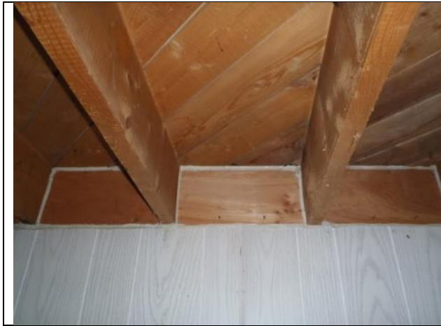
Photo 12 – Blocking over supports
