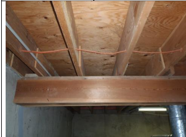
Photo 43 – Main floor joists over central beam
