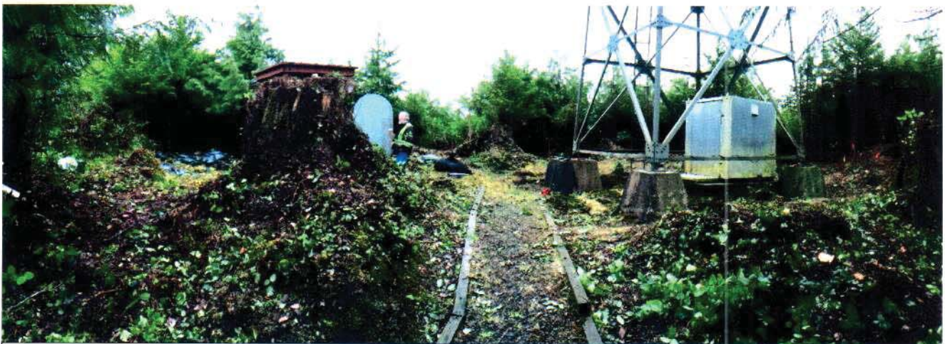
Photo 3 – Existing light tower area looking eastward from gravel path
