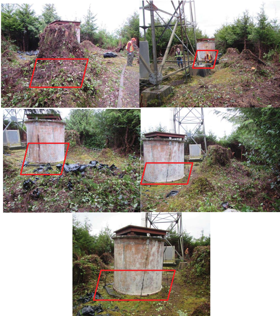
Figure 3: Relocation of Light Tower
