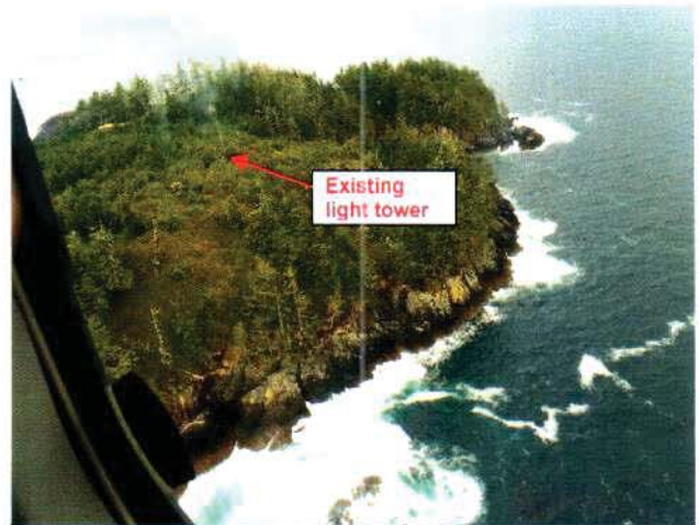
Photo 2 – Existing light tower looking southeastward
