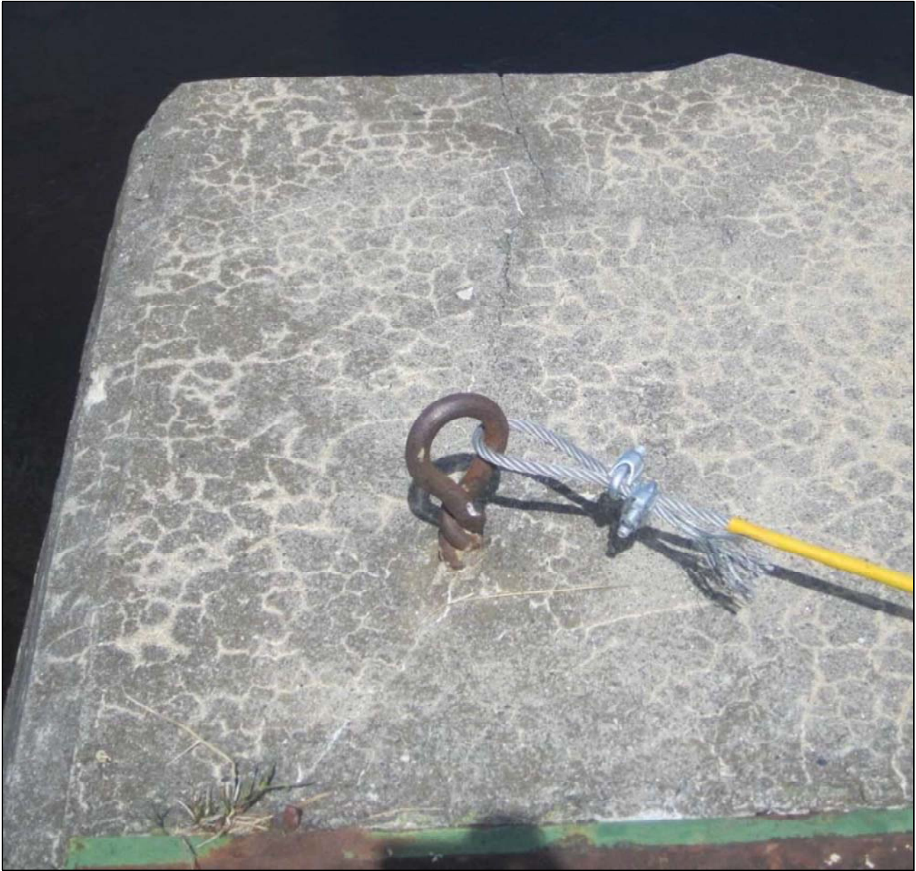
Figure 24: Existing anchor at Portage Dam, right side. Illustration provided to show general configuration only: the new waterway barrier must be upstream of this, and the configuration of wire rope clips is not acceptable.
