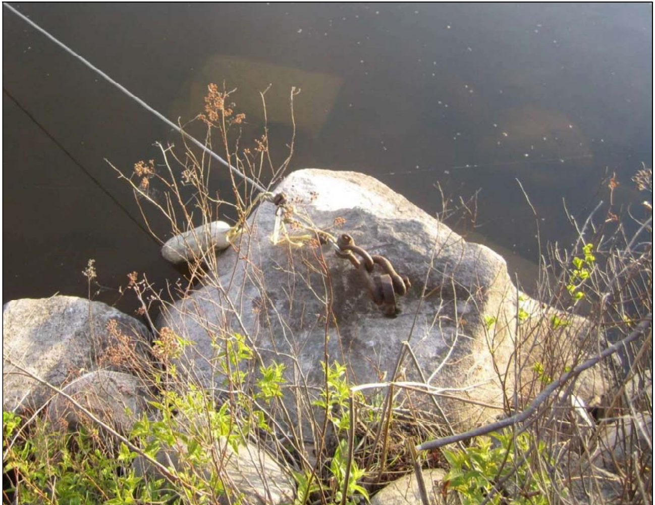
Figure 6: Timiskaming Dam, existing left anchor of existing waterway barrier.
