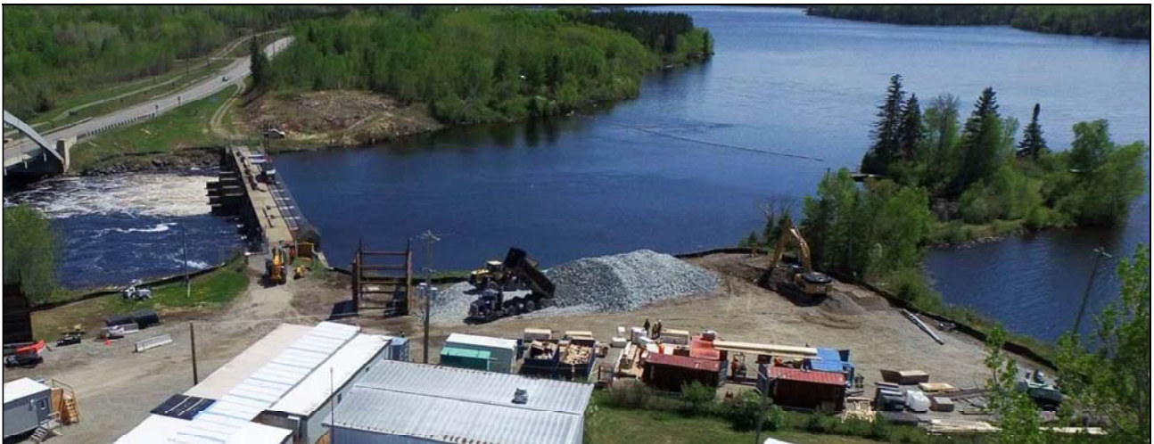
Figure 15: Aerial view of Latchford Dam at start of new dam construction (image from Google Maps). Waterway barrier visible. There is access to left anchor on spit of land via a pathway about wide enough for a pickup truck.
