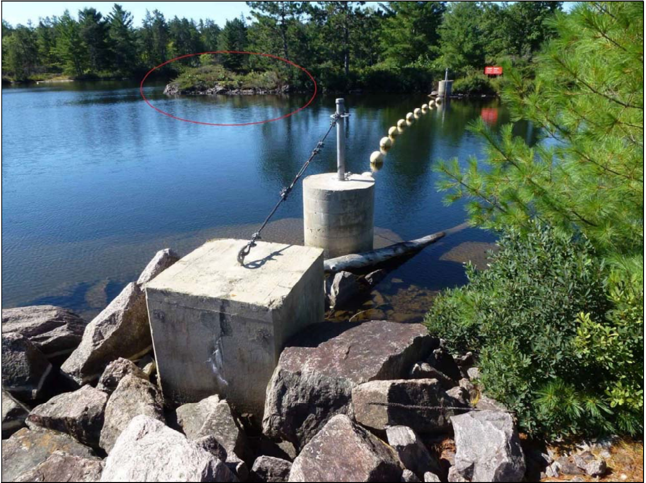
Figure 29: Portage Dam: existing waterway barrier. Area circled in red is approximate location of left anchor of new waterway barrier; detail in next photo (despite the curvature of the existing waterway barrier in this photograph, water flows from left to right in this photograph,).
