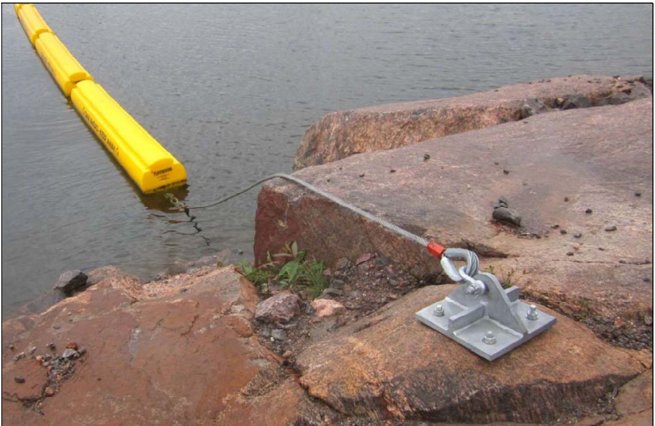
Figure 31: End anchor for the waterway barrier at the Okikendawt Generating Station adjacent to Portage Dam. Photo provided for background information on local conditions.
