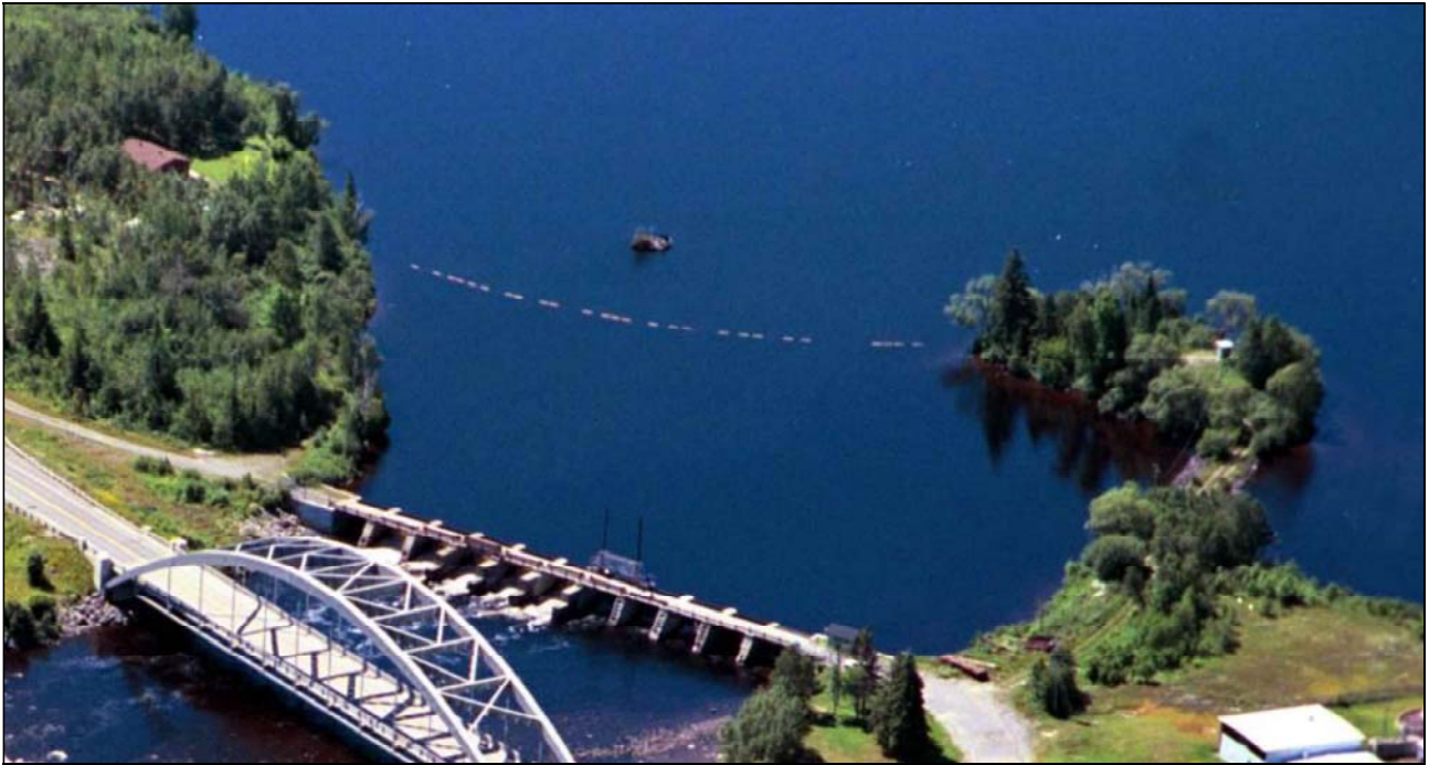
Figure 9: Latchford Dam showing old dam and old waterway barrier (photo taken 2001). New Latchford Dam has been built slightly upstream of the old dam. New waterway barrier to be in similar location as old waterway barrier, with right anchor being placed slightly downstream of existing anchor.
