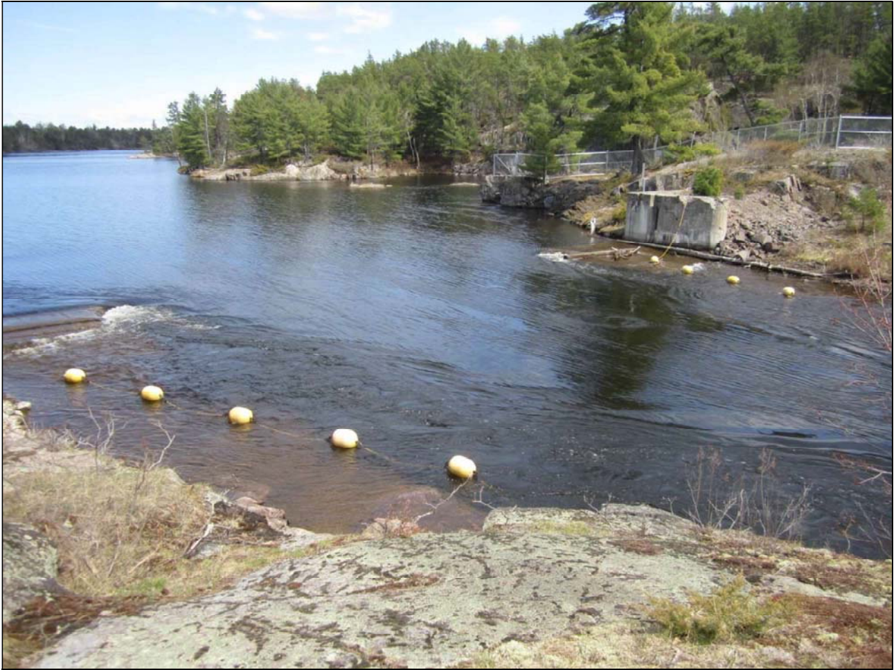
Figure 23: Little Chaudière Dam: area around existing waterway barrier, which was broken at the time the photograph was taken.
