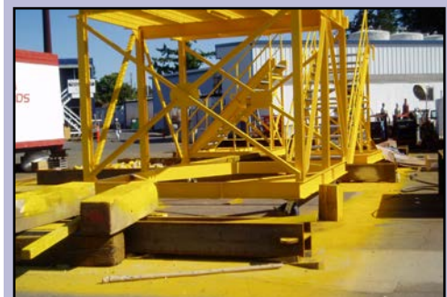
INADEQUATE containment.
