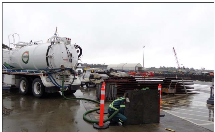
Lift Station Maintenance.
