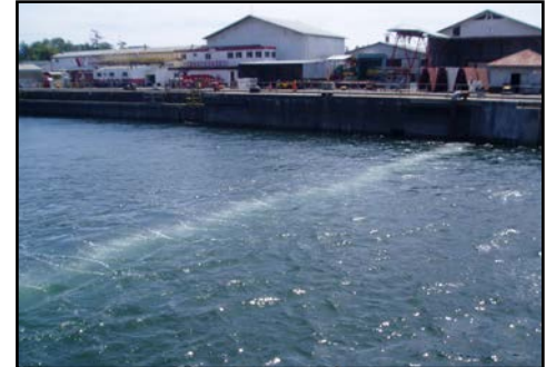
Bubble curtain employed during vessel transfer.
