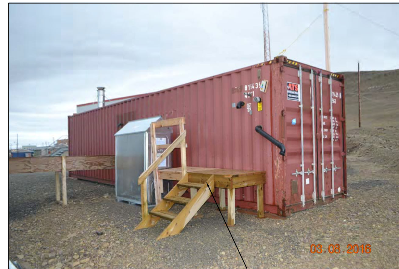
2 PHOTO 1 - PLATFORM - MECHANICAL ROOM A4.1 SCALE: N.T.S.
