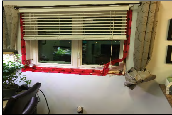
Photo #8 – Kitchen window in Building A.
