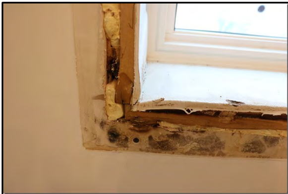
Photo #5 – Mould and water damaged MDF sill on kitchen window of Building B prior to assessment.
