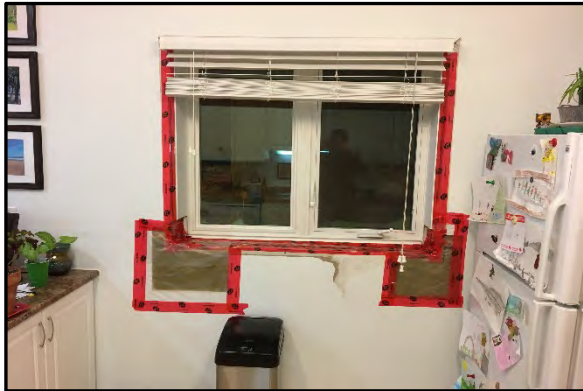
Photo #9 – Kitchen window in Building B.
