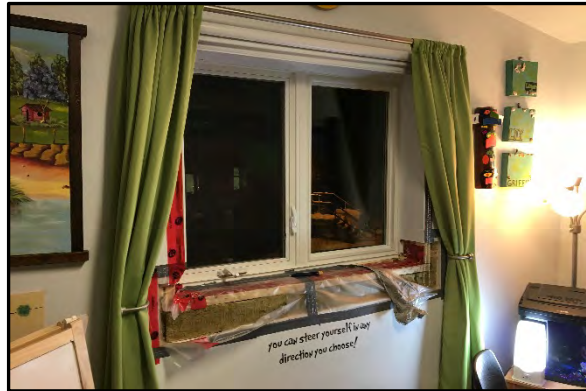
Photo #10 – Bedroom 2 window in Building B.
