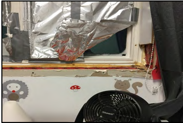
Photo #7 – Bedroom 3 window in Building A.
