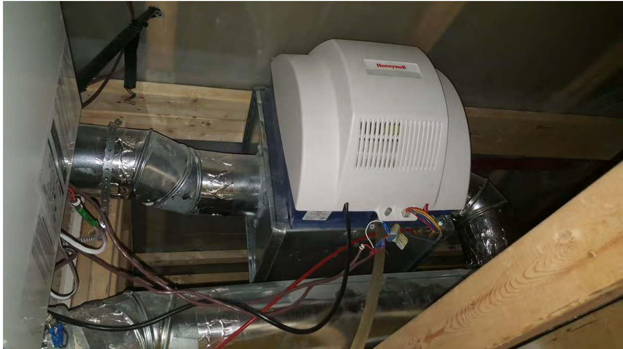
Photo 3 Existing Humidifier
