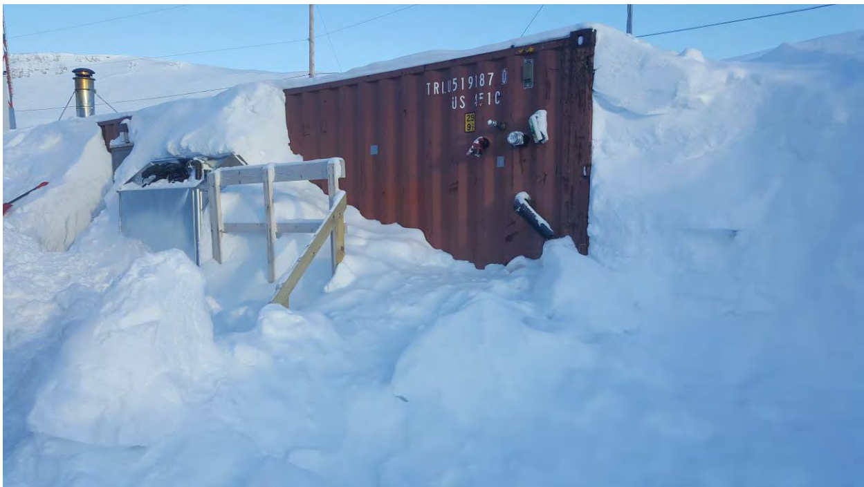
Photo 18 - Exterior Fuel Tank
