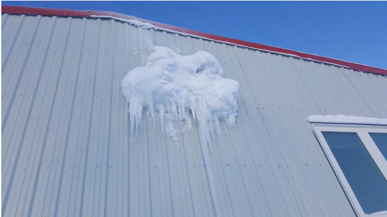
Photo 7 Existing Exhaust and Supply Outlets
