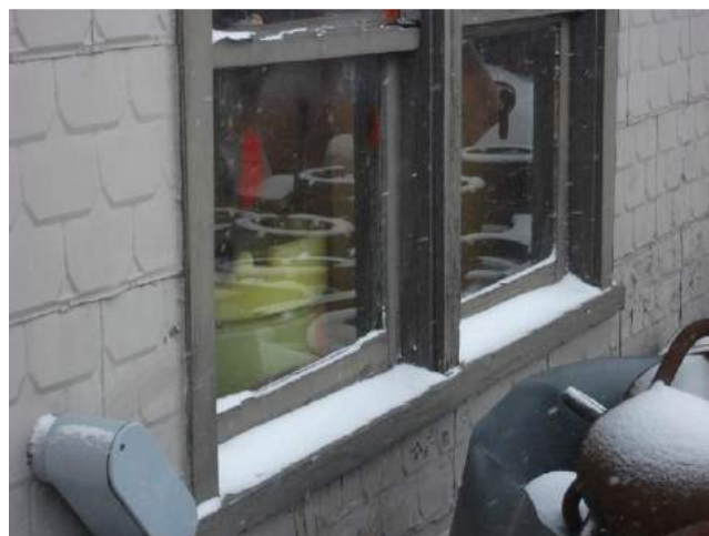
Photograph 32: Boat House Building – Lead-Based Green Exterior Window Paint
