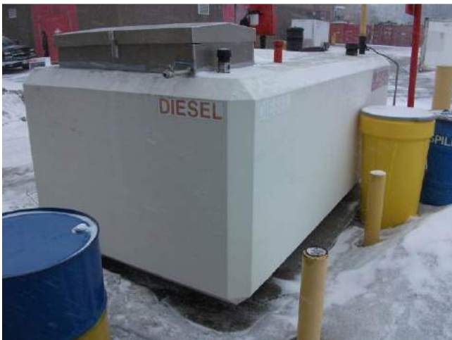
Photograph 23: Helicopter Hangar Building – Diesel Fuel Storage Tank
