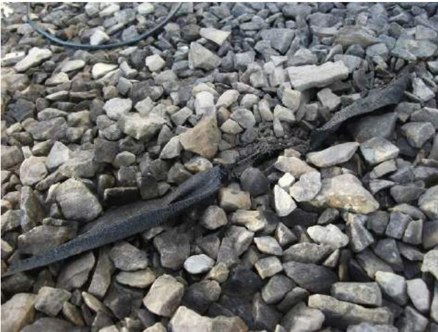
Photograph 7: Roof Ballast Filter Fabric/Cloth on the Roof of the Main Building at CCGB Prescott
