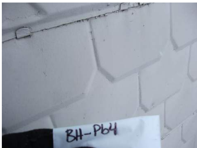
Photograph 31: Boat House Building – Lead-Based Beige Exterior Wall
