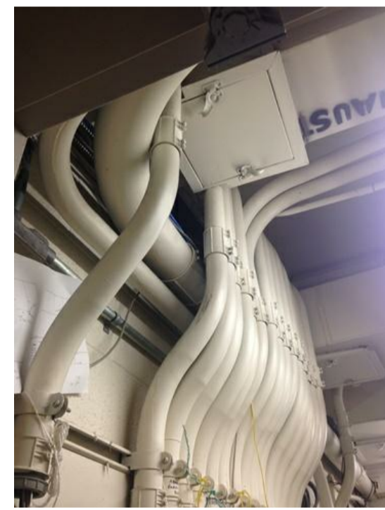
ROOM 212 & 213 - JANITOR & CORRIDOR PHOTO 262
