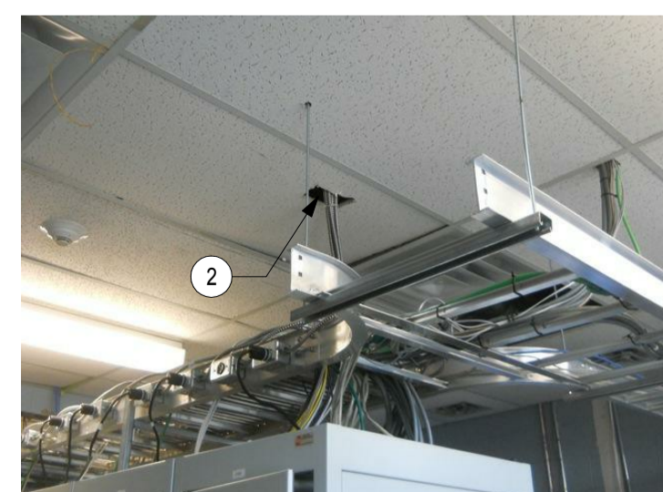
ROOM 007 - YARD OFFICE PHOTO 105
