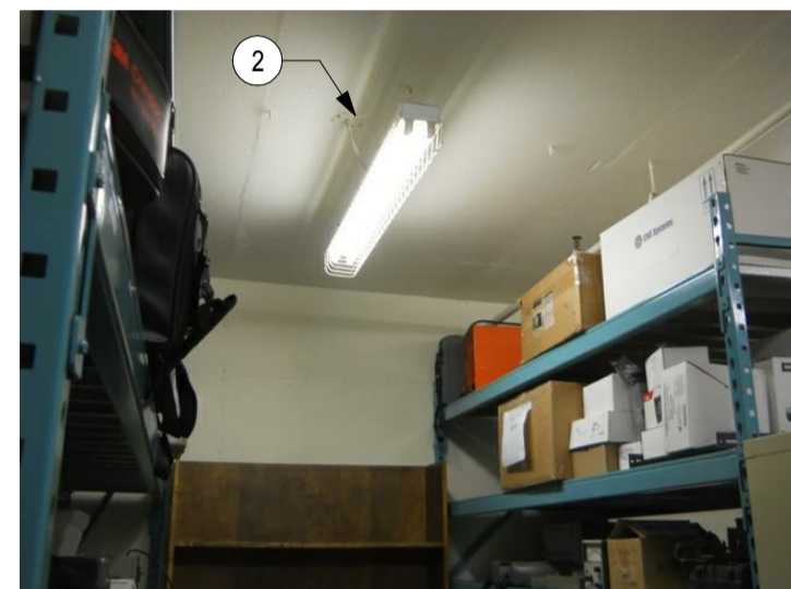
ROOM 010 - T & E WORKSHOP PHOTO 118
