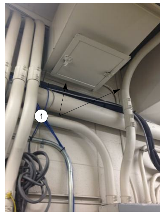
ROOM 212 & 213 - JANITOR & CORRIDOR PHOTO 256
