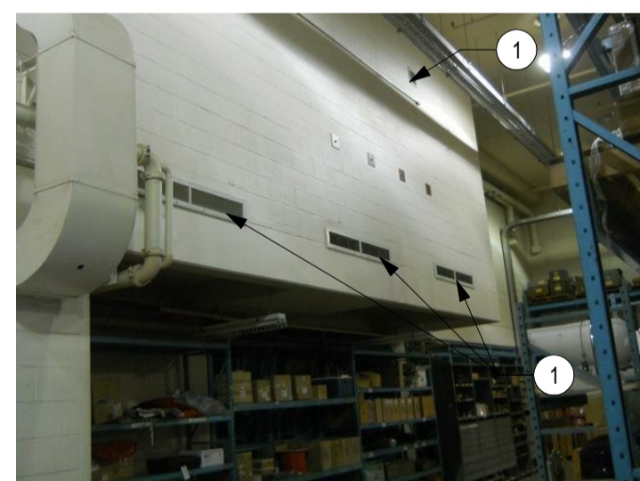
ROOM 019 - SHIPPING & RECEIVING PHOTO 166
