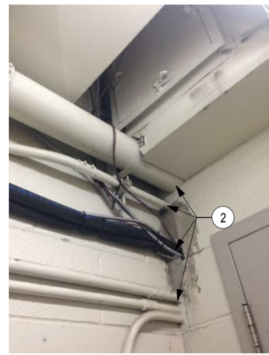
ROOM 212 & 213 - JANITOR & CORRIDOR PHOTO 257
