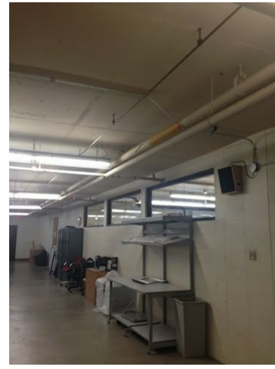
ROOM 104 - MEZZANINE STORAGE PHOTO 224
