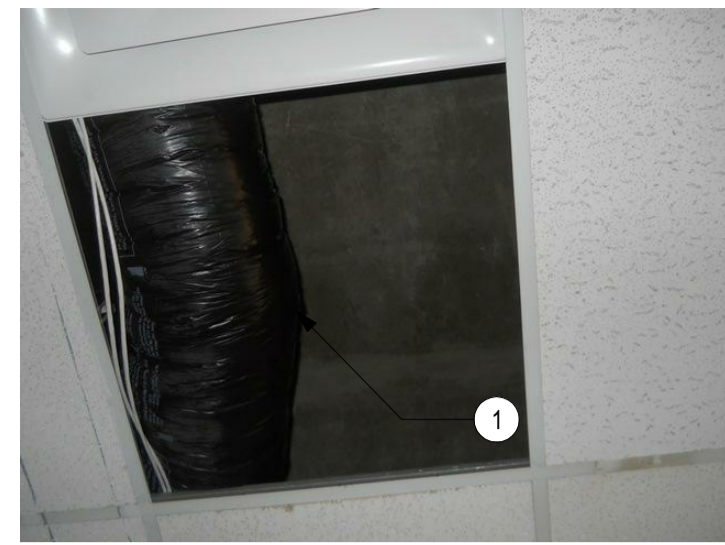
ROOM 007 - YARD OFFICE PHOTO 108
