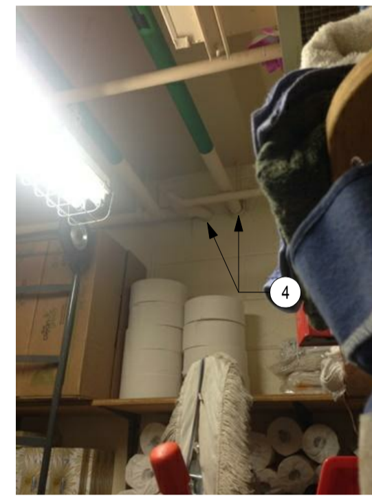
ROOM 019 - SHIPPING & RECEIVING PHOTO 189
