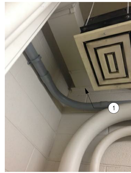
ROOM 212 & 213 - JANITOR & CORRIDOR PHOTO 254
