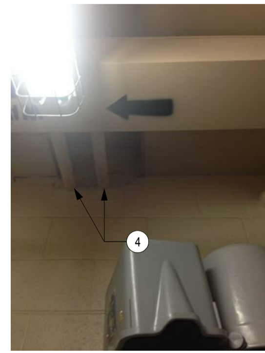
ROOM 019 - SHIPPING & RECEIVING PHOTO 187
