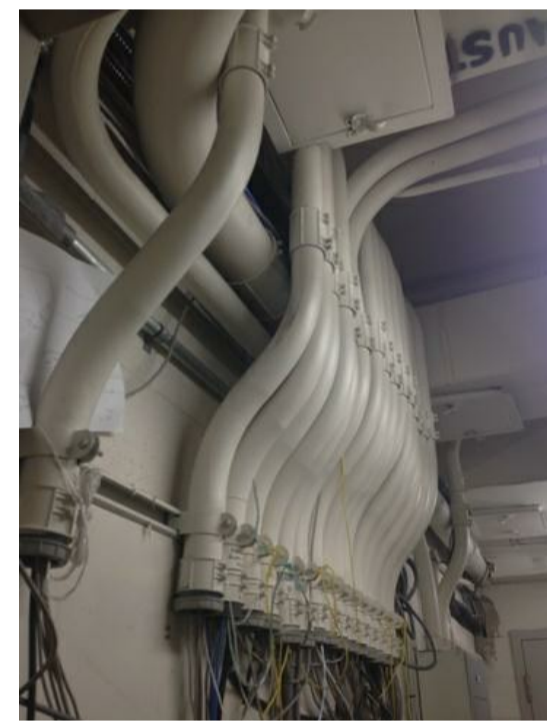
ROOM 212 & 213 - JANITOR & CORRIDOR PHOTO 261
