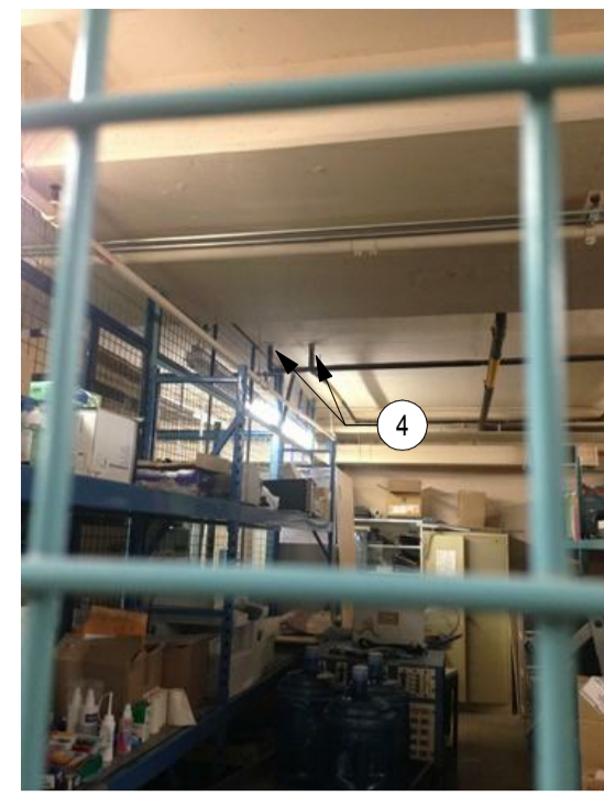
ROOM 125 - ILLUMINATION WORKSHOP PHOTO 242
