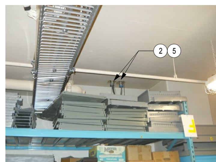
ROOM 019 - SHIPPING & RECEIVING PHOTO 172
