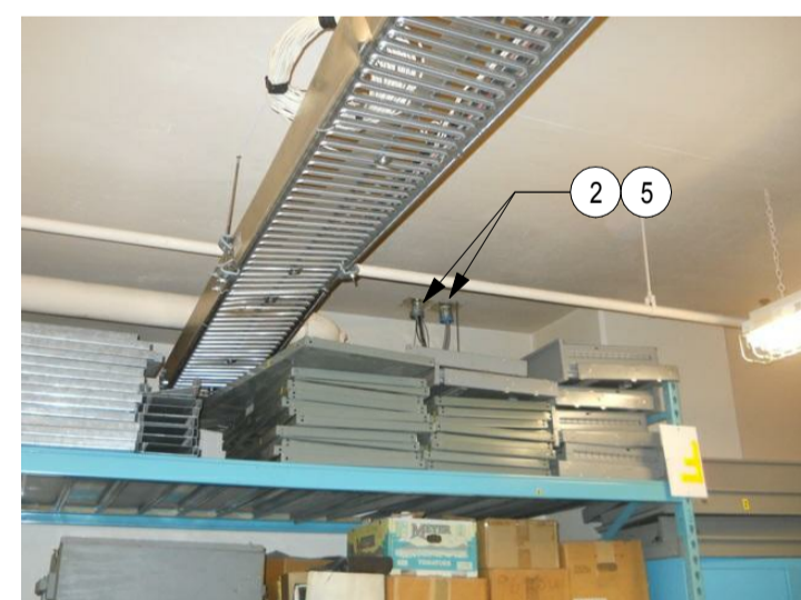
ROOM 019 - SHIPPING & RECEIVING PHOTO 171
