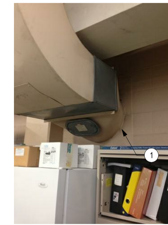
ROOM 125 - ILLUMINATION WORKSHOP PHOTO 237
