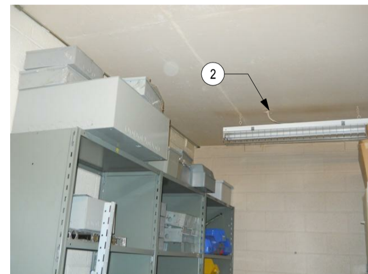
ROOM 011 - OFFICE 014 PHOTO 122
