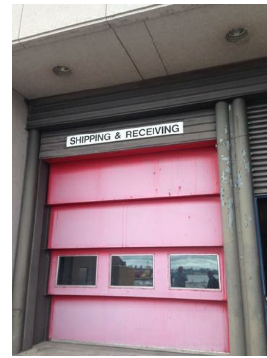
ROOM 019 - SHIPPING & RECEIVING PHOTO 184
