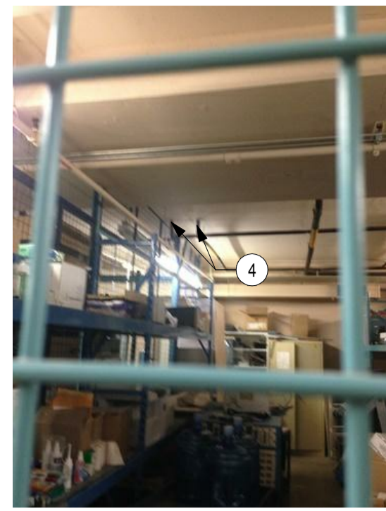
ROOM 125 - ILLUMINATION WORKSHOP PHOTO 241
