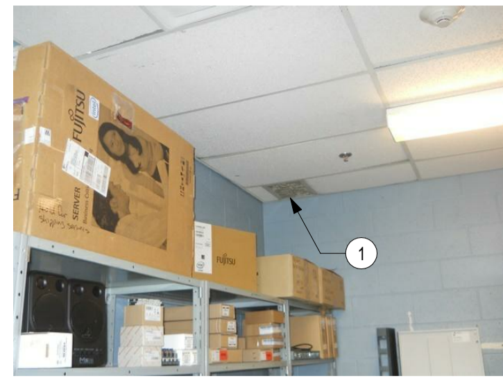
ROOM 007 - YARD OFFICE PHOTO 107
