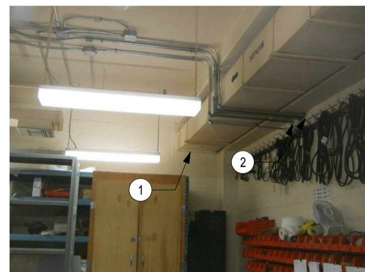
ROOM 011 - OFFICE 014 PHOTO 125
