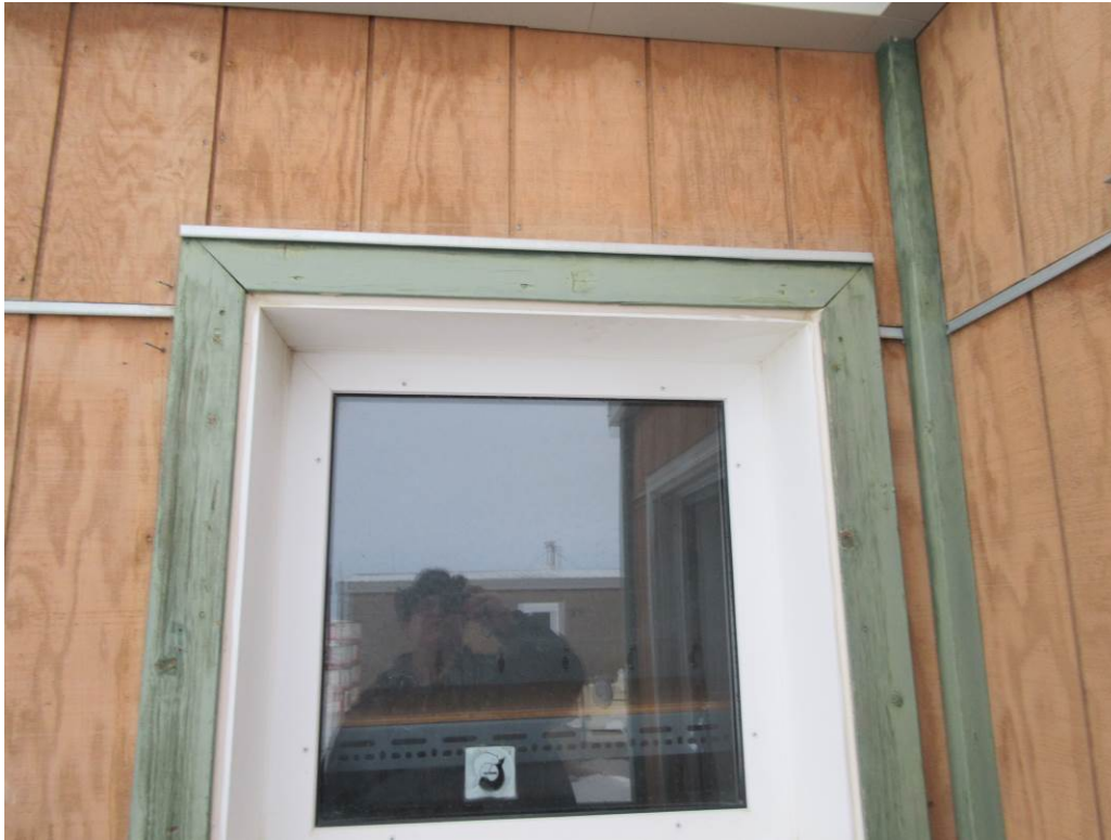
Photo 13 Typical Exterior Window
