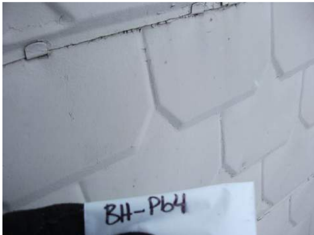
Photograph 31: Boat House Building – Lead-Based Beige Exterior Wall
