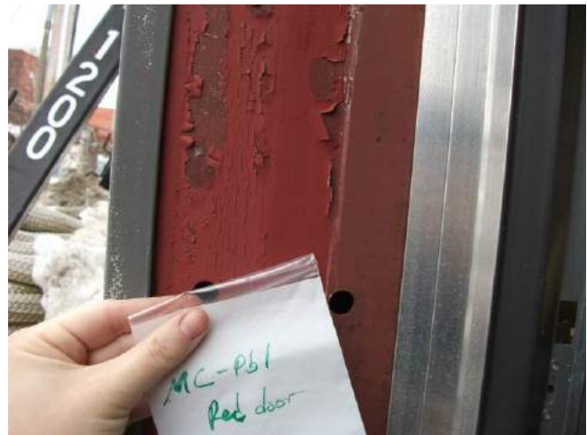
Photograph 12: Metal Clad Storage Building – Lead-Based Red Door Paint
