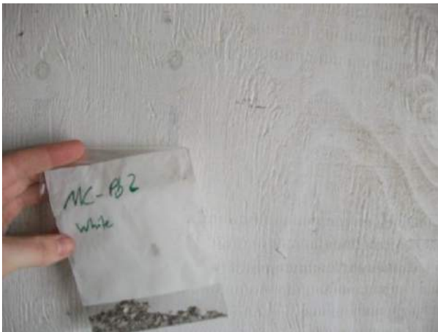
Photograph 11: Metal Clad Storage Building – Lead-Based White Wall Paint
