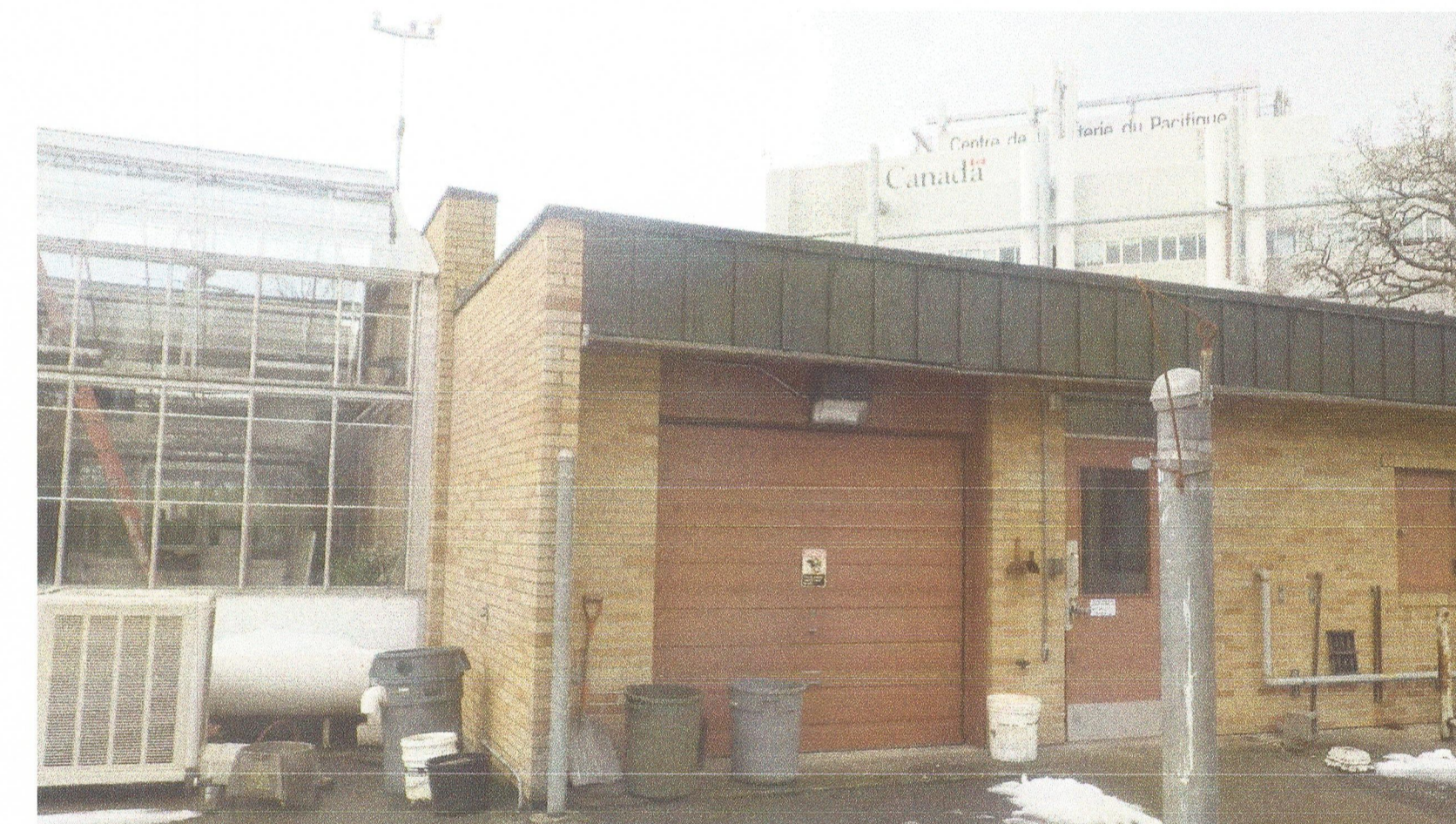
4 PHOTO OF EXISTING EAST ELEVATION BE1.2 NTS
