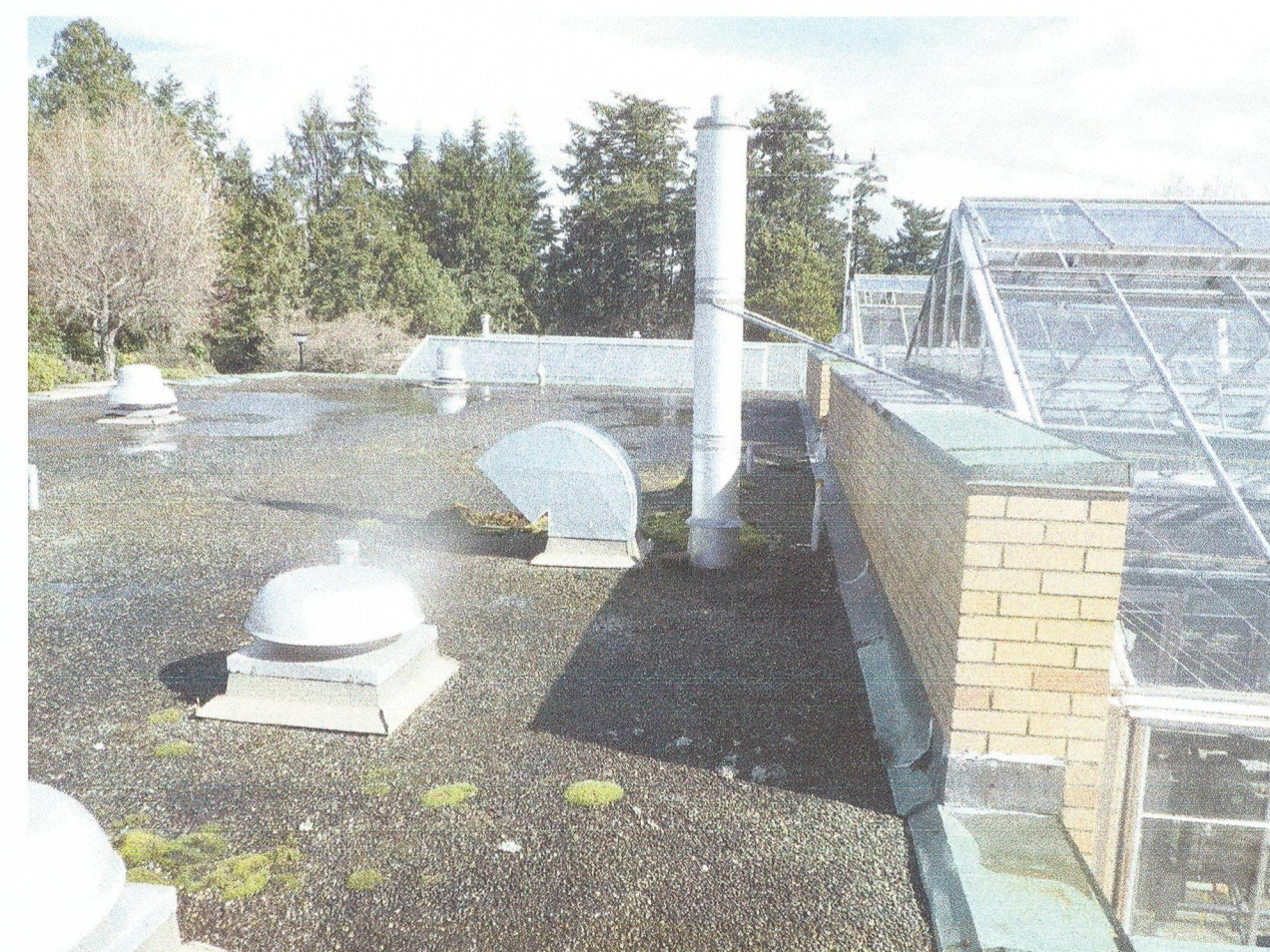
5 EXISTING ROOF PHOTO AT SOUTH-EAST CORNER BE1.2 NTS
