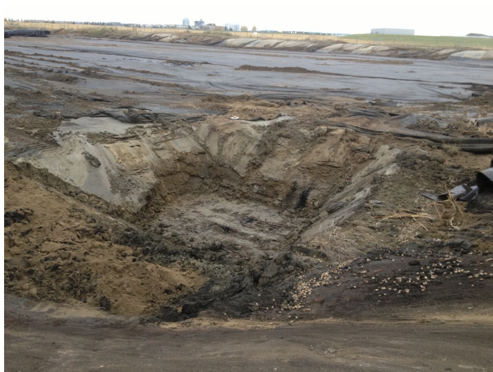
Photograph 8: North sump prior to backfilling.
