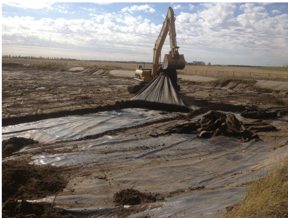
Photograph 9: Removing the top geotextile liner.
