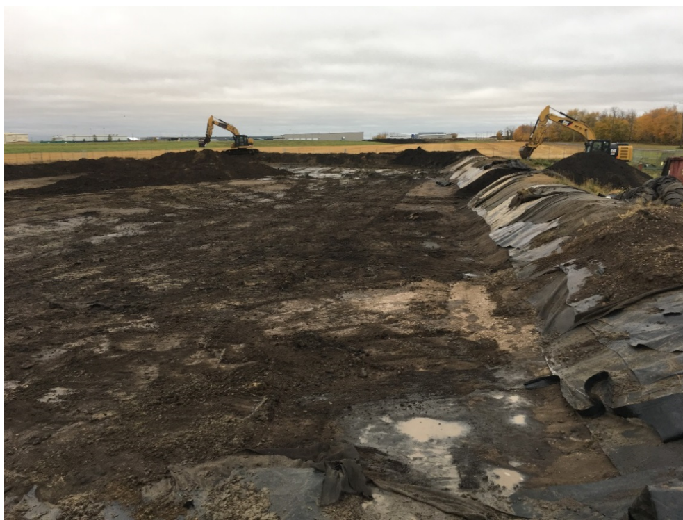
Photograph 11: Removing the liner from the berm and spreading soil in the north cell.
