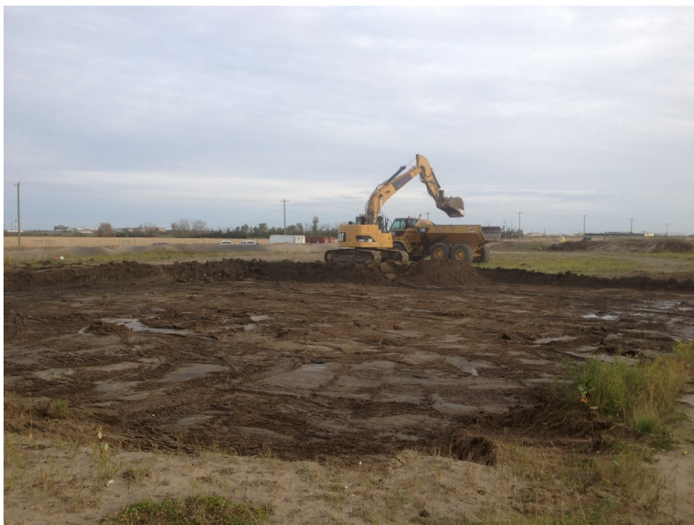
Photograph 6: Removing soil from the north cell.
