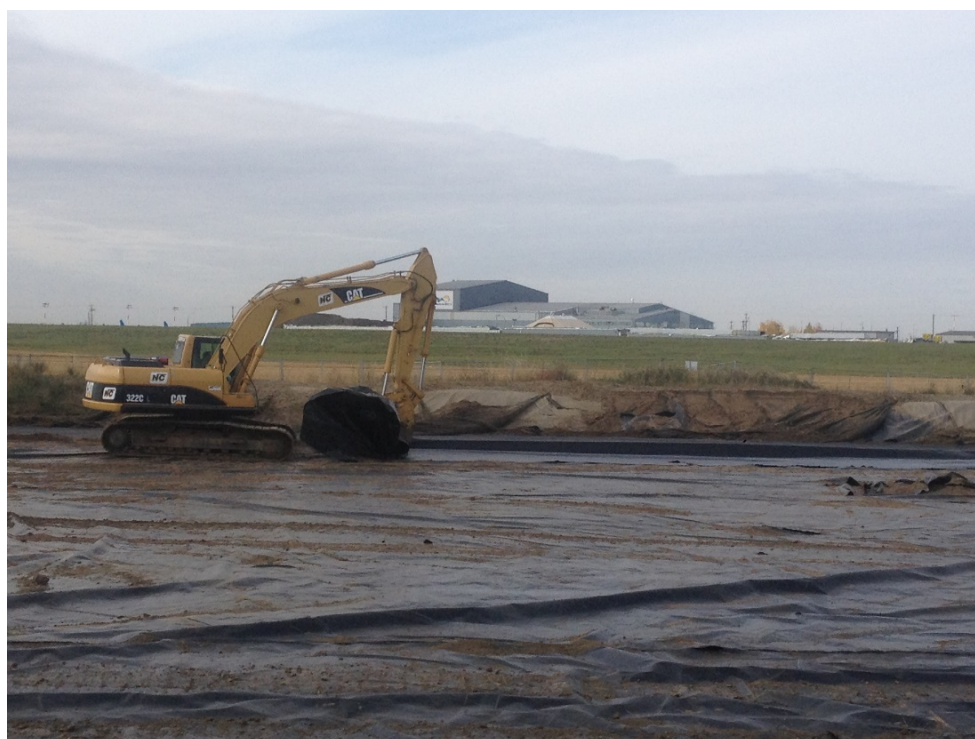
Photograph 10: Removing the second liner.
