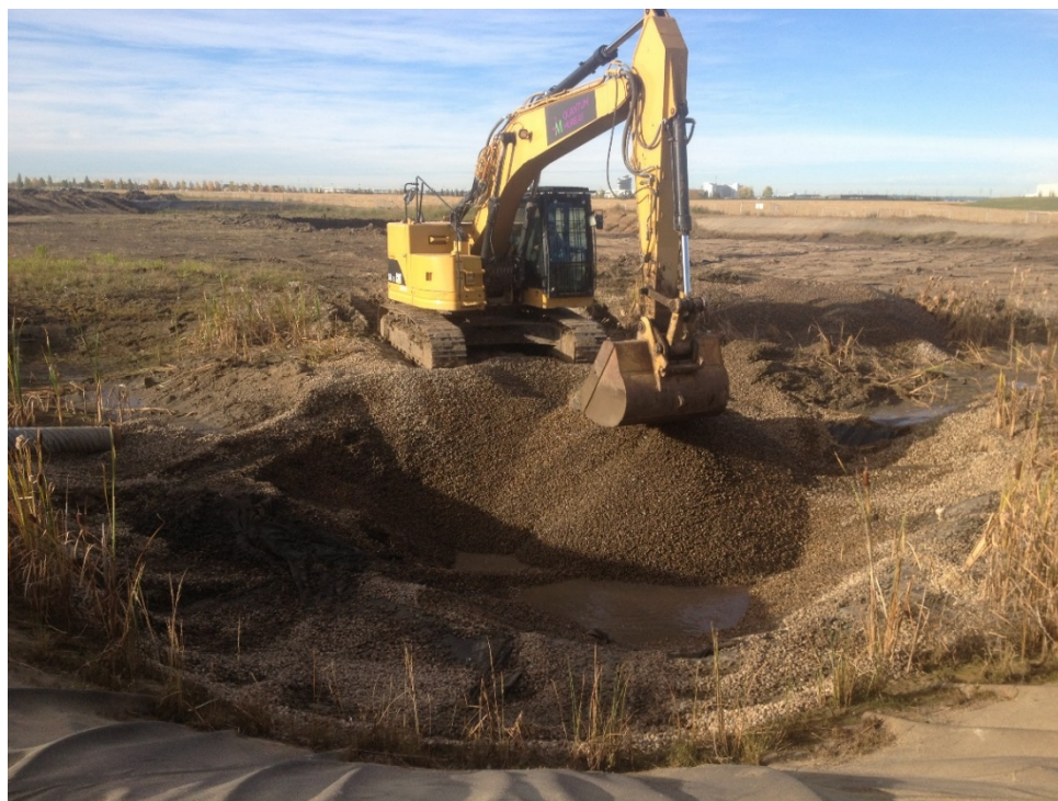
Photograph 7: Removing gravel from the north sump.
