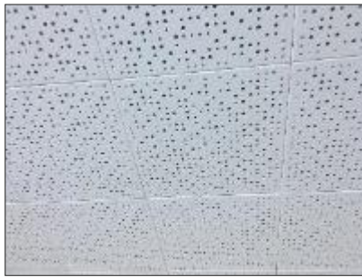
Photograph No. 4 – 12" x 12" wood fibre ceiling tiles in the Souris detachment.
