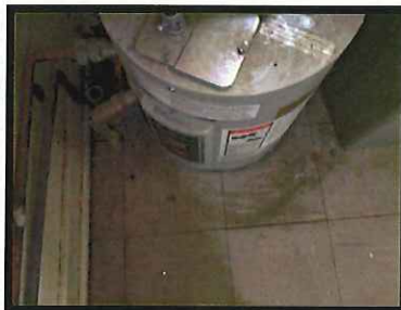
Photo Set 2 Building 28 - Asbestos containing 9"x9" tan vinyl floor tiles within the office area washroom
