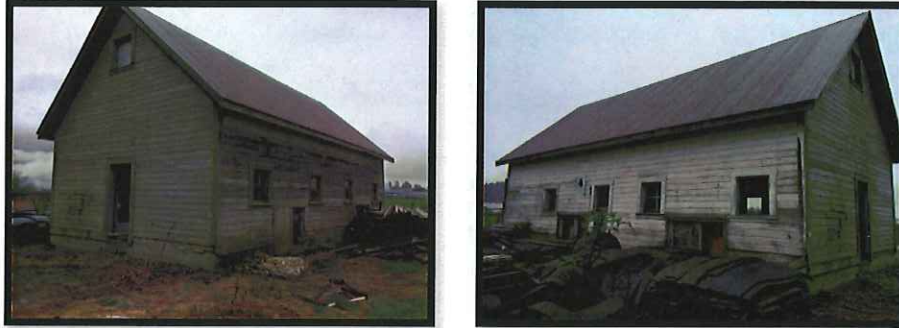
Photo Set 5 Building 50 – The Piggery (Farm Structure) Exterior
