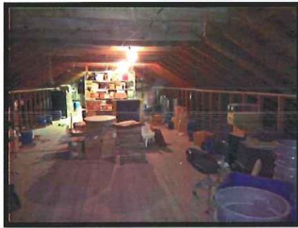
Photo Set 3 Building 28 – Asbestos-containing vermiculite attic insulation
