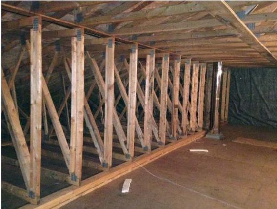
The problem is a lack of anchorage back to the original structure, and from piggyback trusses to lower trusses. The lower (not piggyback trusses) were placed on 2x6 timber plates. There are either 1, 2 or 3 layers of plates depending on location. Additional shimming of plates was done also making for a maximum height of approximately 6" at drain locations.
