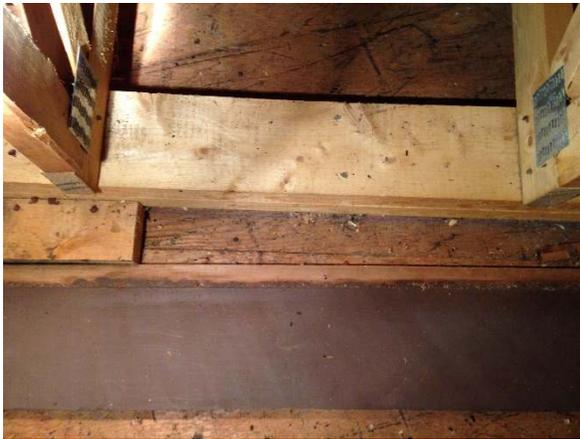
The timber plates are nailed down to the plywood sheathing generally with 2 nails every 16" to 24". The main trusses are nailed down to the plates with either 2 or 3 nails. At quite a few locations the bottom chord is split from improper nailing.
