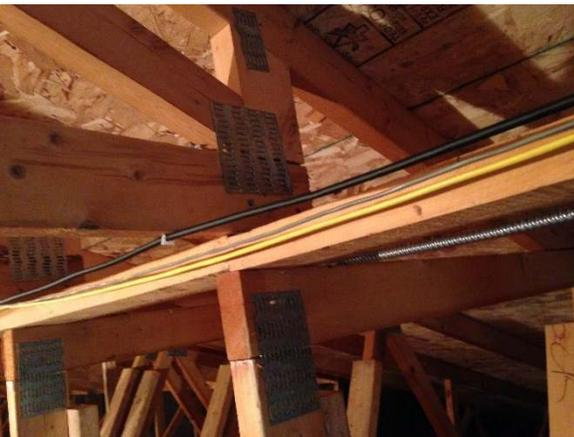
The piggyback trusses bear on top of the main trusses with either a 1x4 or 2x4 separating them. The upper piggy back trusses are only nailed down to the plate with no direct connection between the trusses.
