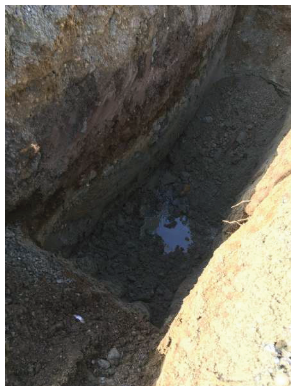
Photo 2: Looking into TP16-01, note fill near surface and the minor water seepage pooling at the bottom.
