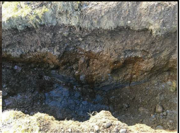
Photo 5: Looking into TP16-04, note water seepage from below the fill in the sand and gravel soil unit.
