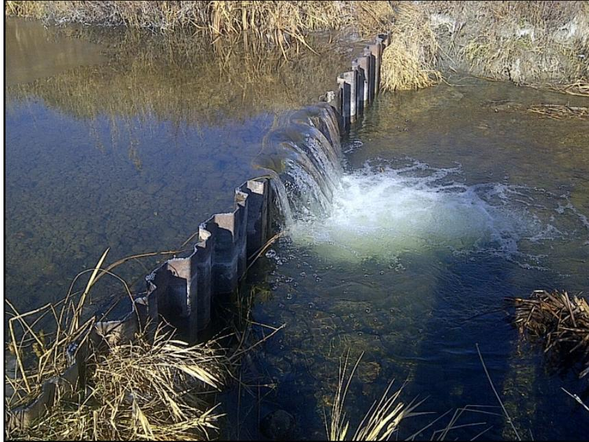
*Photograph 7: Typical steel sheet pile weir.*
