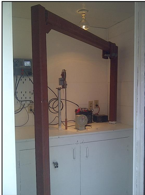
*Photograph 6: Fall restraint anchor frame inside a shelter on a well.*
