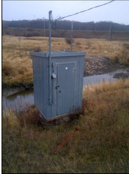
*Photograph 5: Typical shelter on top of a creosote well*
