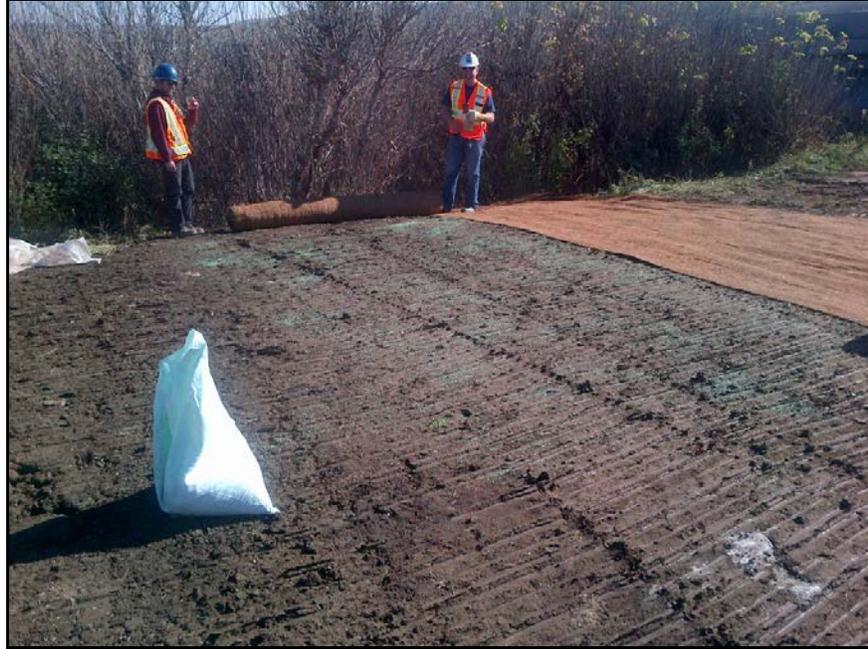
*Photograph 9: Erosion control matting placed over compacted disturbed soil and native seed.*
