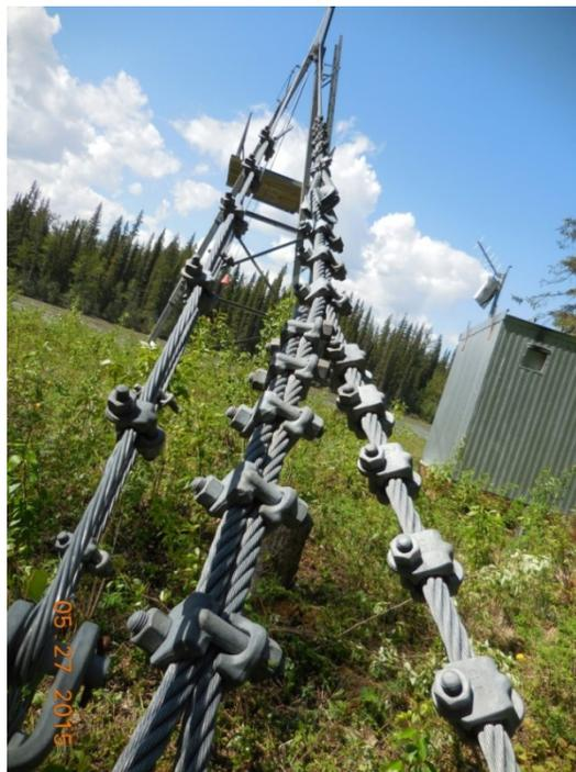
*Photograph 4: Typical clip-type cable terminations.*
