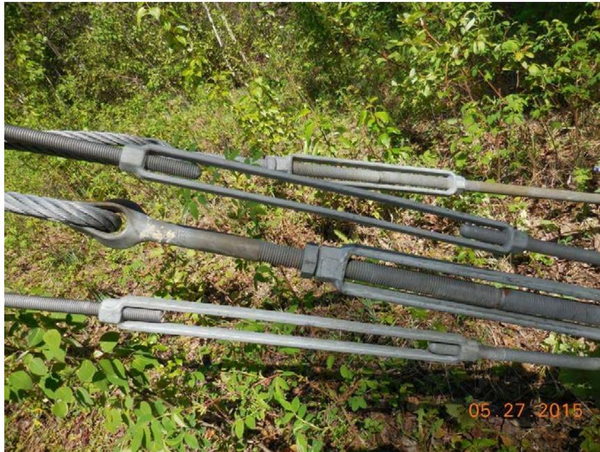
*Photograph 3: Typical cable turnbuckle arrangement.*
