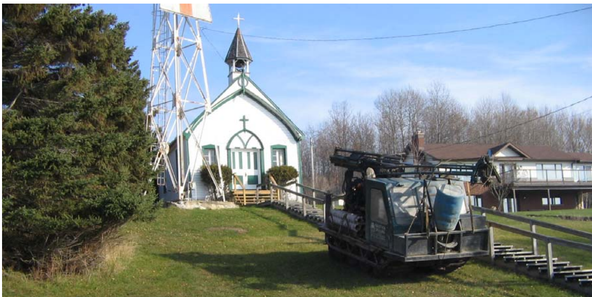
Photo 2: Mobilizing drill rig to borehole location.
