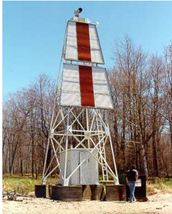
Photo 1: Existing Hay Point Rear Range tower.
