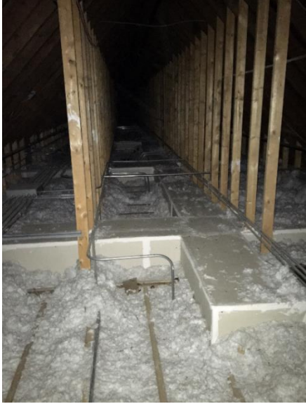
Q9, Photo 1-attic bulkheads
