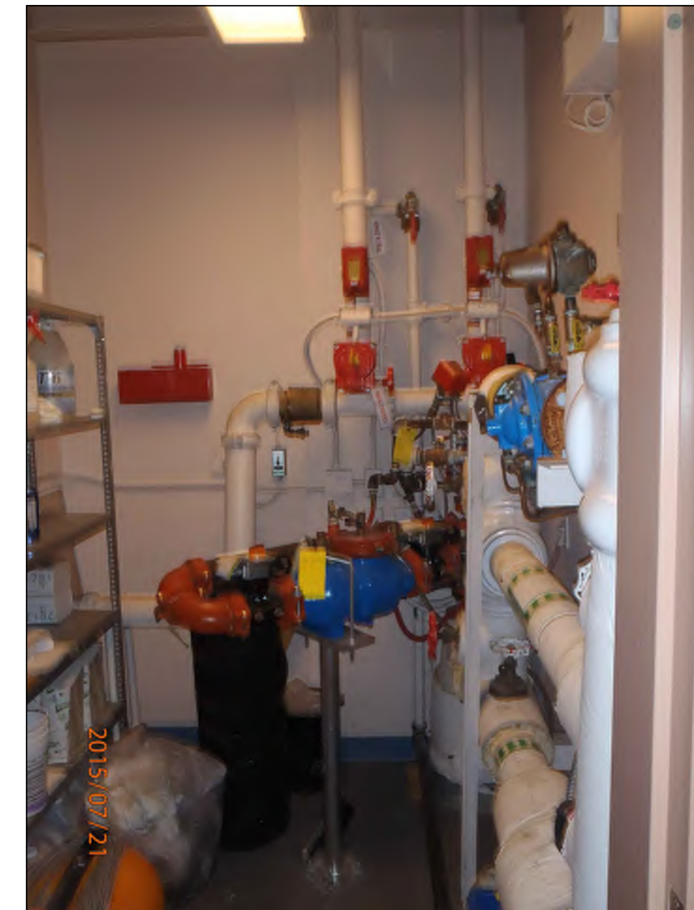
EXISTING SPRINKLER VALVE STATION N.T.S.
