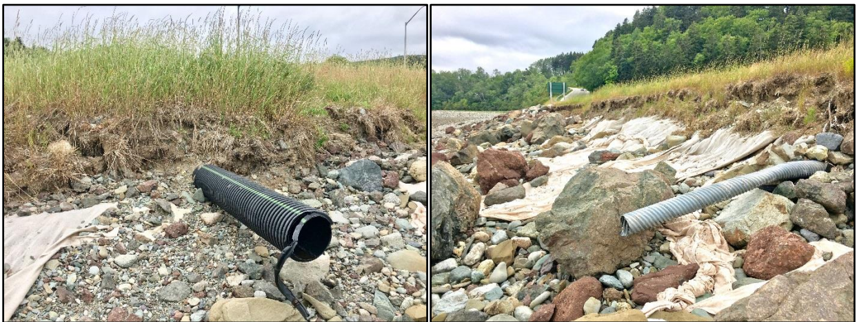
Figures 13-14: View of the exposed corrugated drainage pipes and fabric layers
