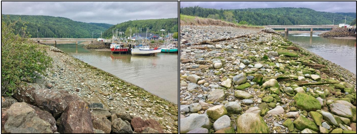
Figures 7-8: View of the old cribwork along the Upper Salmon River
