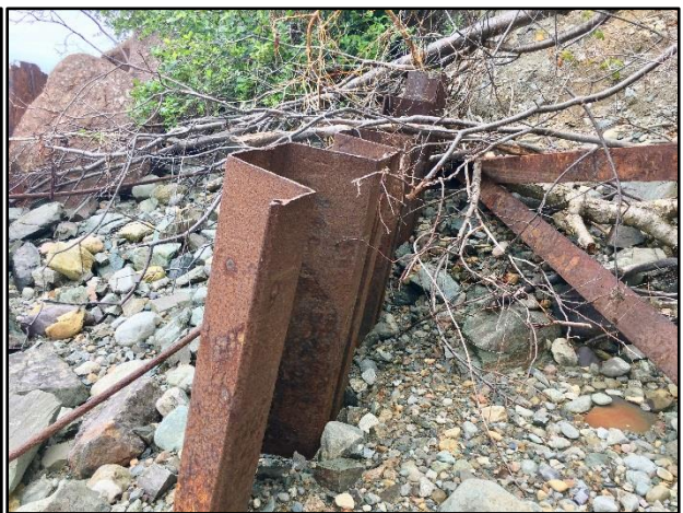
Figures 24-25: View of the deteriorated steel sheet piling
