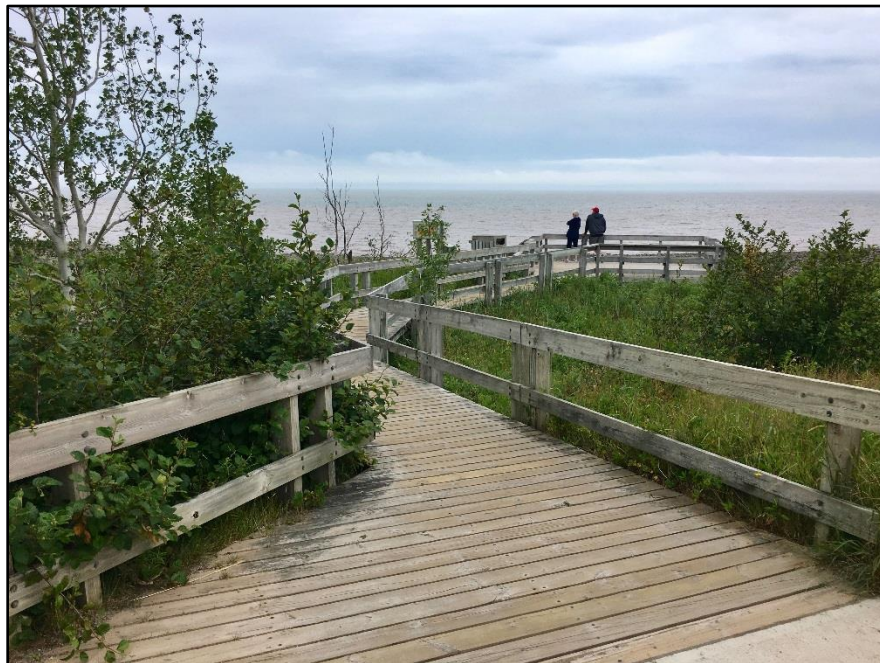
Figure 9: View of the walkway and deck facing the Bay of Fundy
