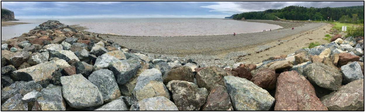
Figure 3: Panoramic view of the project location from the breakwater
