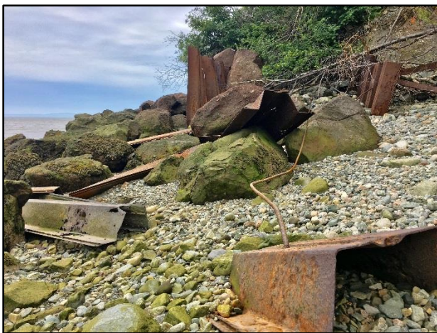
Figures 24-25: View of the deteriorated steel sheet piling
