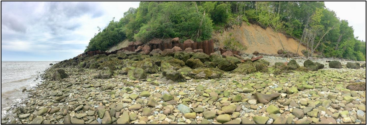
Figure 21: Panoramic view of the armour stone and its steel sheet piling
