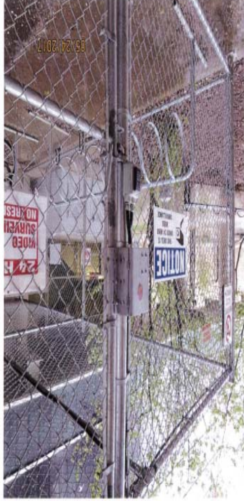
S/W Outdoor bicycle cage card reader and lock release.
