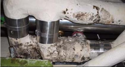
A close-up photograph showing a section of a chiller pipe wrapped in white insulation. The insulation is heavily covered with a thick, dark, fuzzy growth of mould. The pipe itself is metallic and partially visible through the insulation. | 2015                    | Mould on chiller pipe insulation. |
