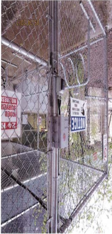
S/W Outdoor bicycle cage card reader and lock release.
