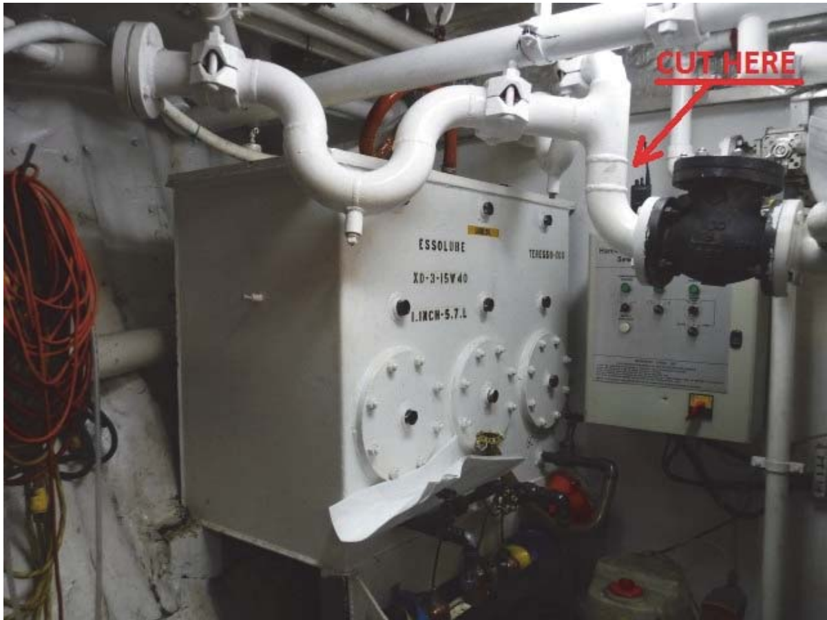
Lube oil storage tank & location of where to splice into existing grey water drain.
