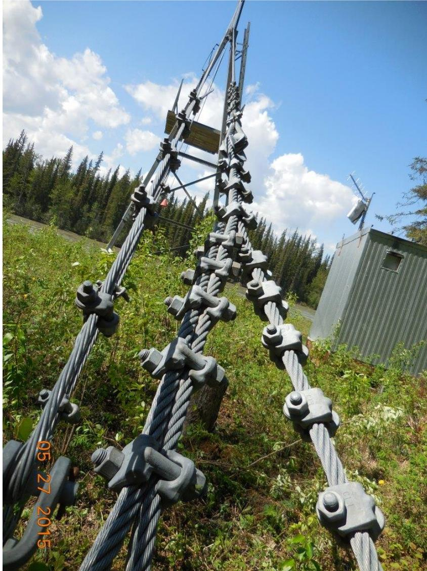
*Photograph 6: Finlay River (above Akie River) “home side” clip-type wire rope end connections.*
