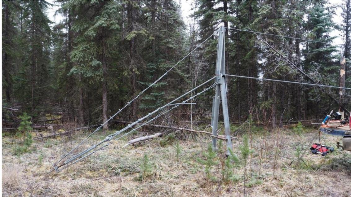
*Photograph 2: Nechako River (below Cheslatta Falls) cableway system, south “home side” tower and tie-back staylines.*
