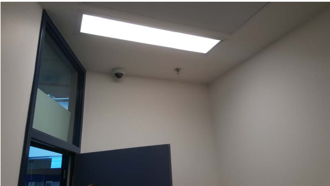
Photo 14 - Window over Door for Room 1-103
