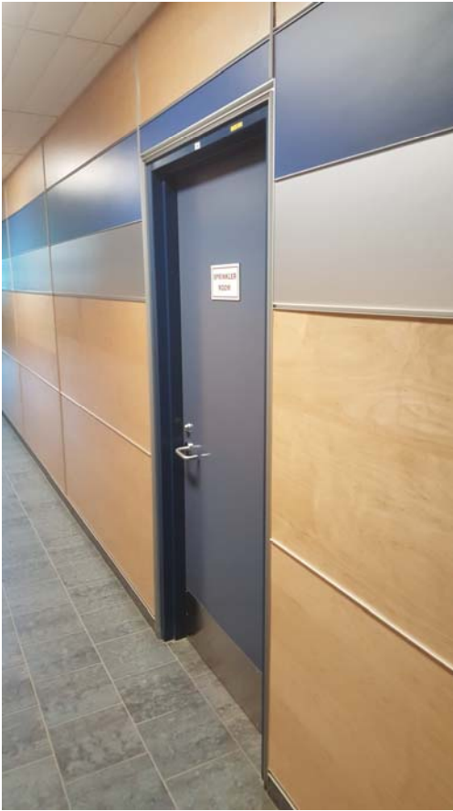
Photo 13 - Typical Hallway Door
