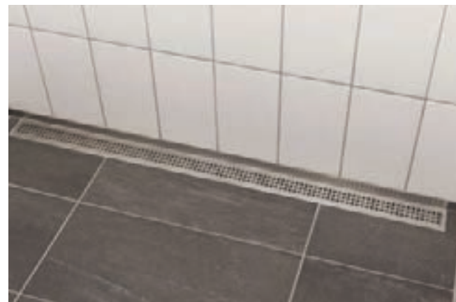
Sample of Linear Floor Drain
