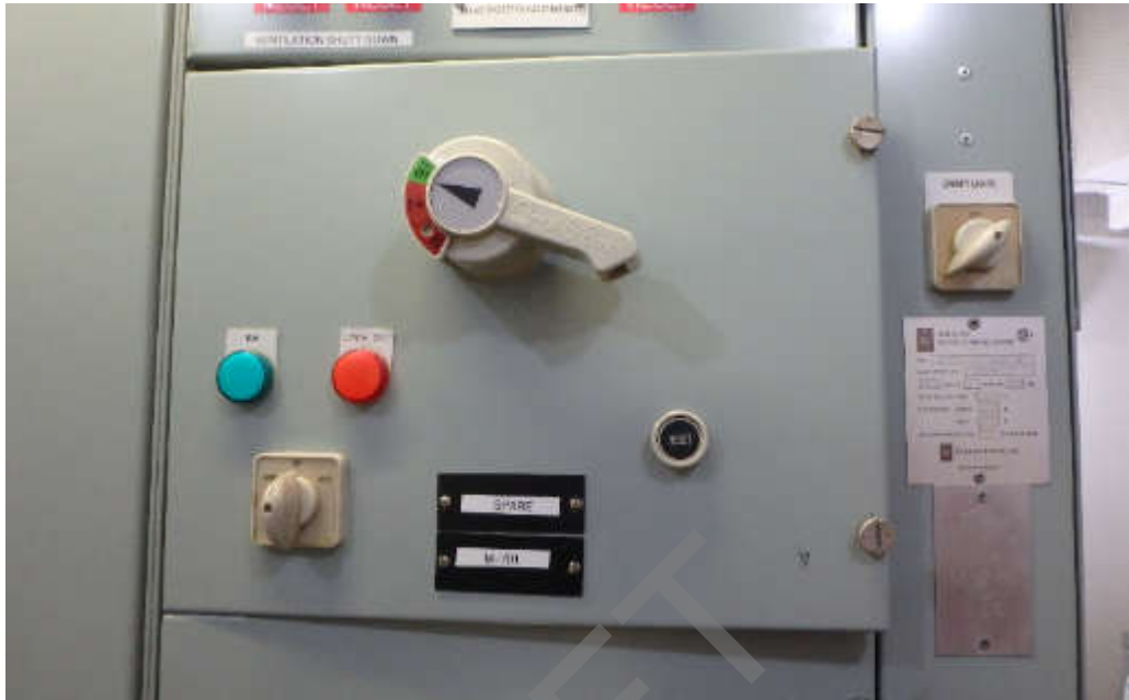
Figure 38 Spare M-701 feeder, in forward equipment room
