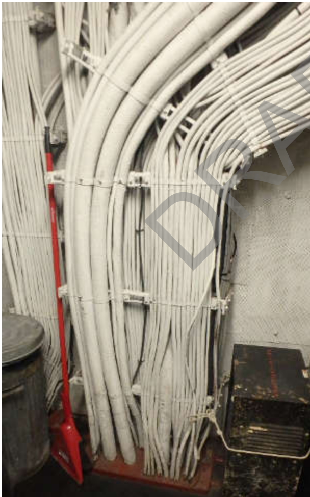
Figure 34: Vertical route in static inverter compartment
