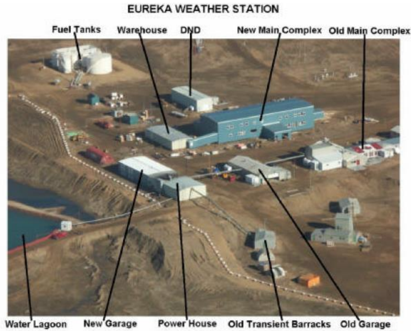
Photo 1 - Aerial View of the Weather Station
