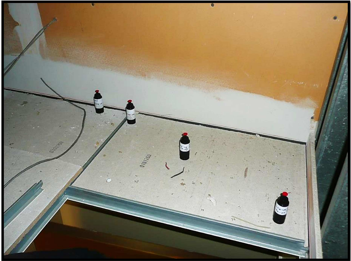
Site sampling location → Room 1217, northwest corner, from on top of the suspended ceiling tile.
