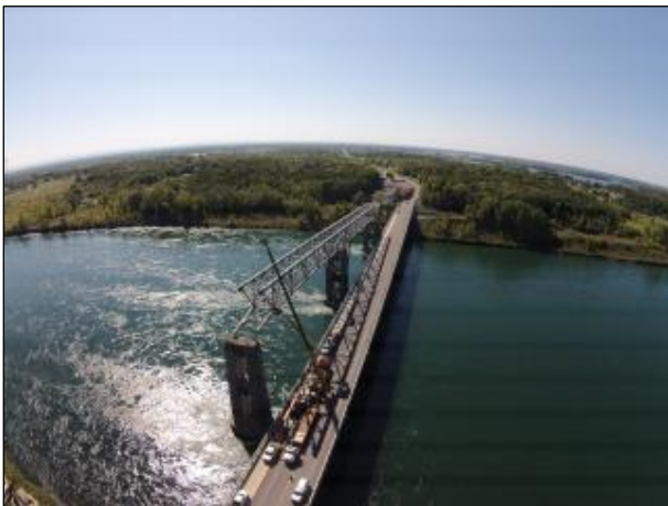
Fig. 2: View of bridges looking South (2015-09-15)
