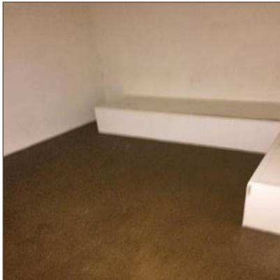
Photo # 5 - Non-asbestos vinyl composite flooring within the cells and corridor.
