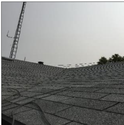
Photo # 6 - Non-asbestos asphalt shingles.
