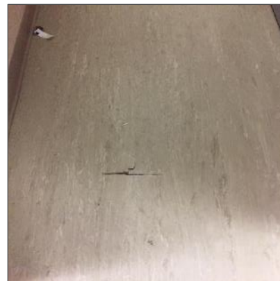
Photo # 4 - Non-asbestos vinyl sheet flooring with paper backing.
