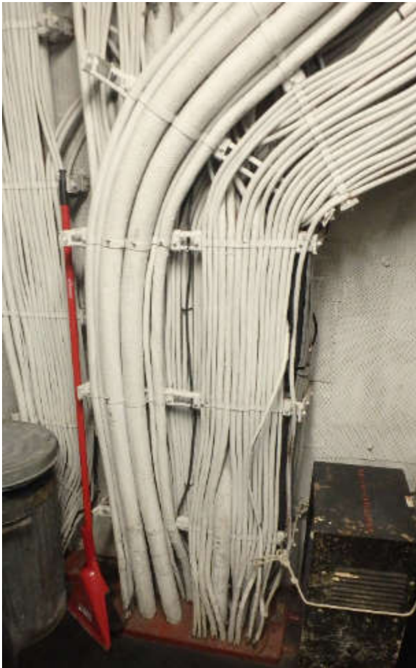
Figure 37 Vertical route in static inverter compartment
