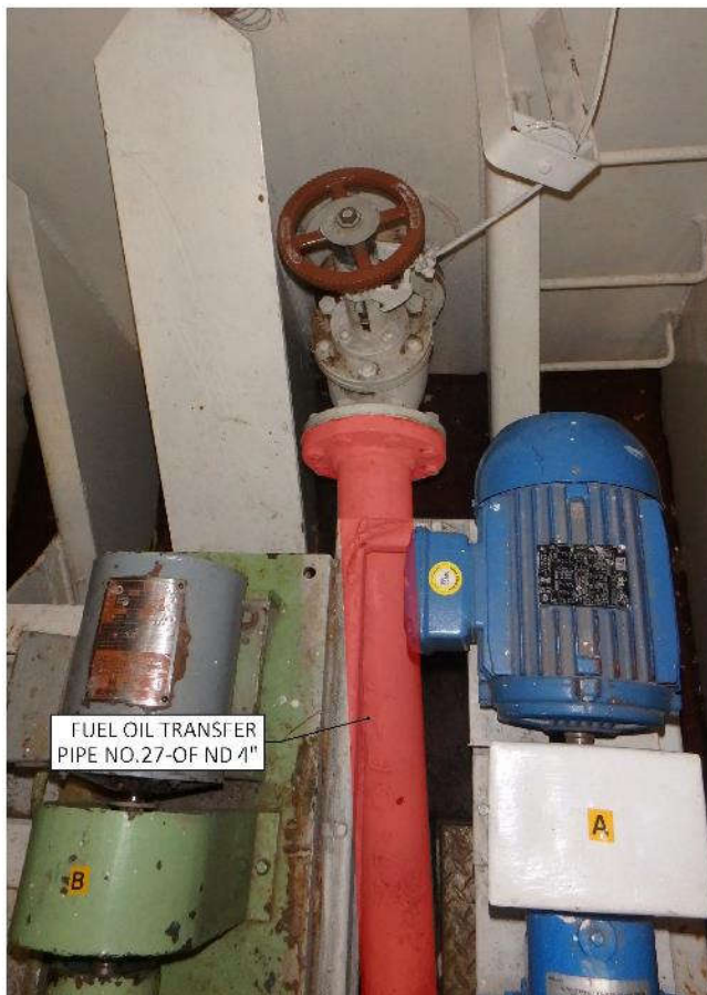
Figure 19 Fuel Oil Transfer 27-OF, connection at longitudinal bulkhead
