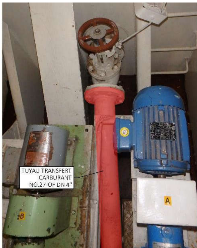
Figure 19 Transfert de carburant 27-OF, raccord à la cloison
