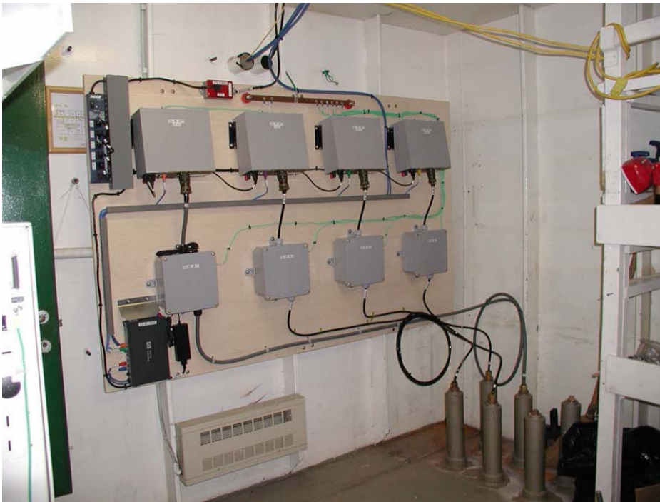
Figure 1. Transceiver units, junction boxes (under GPTs), transducer conduits, cables to the transducer conduits and network switch mounting.
