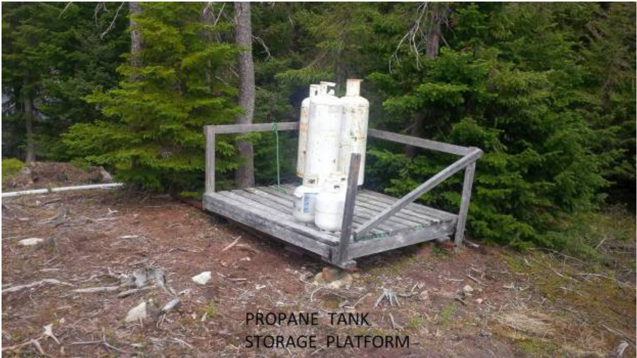
Propane Tank Storage Platform
