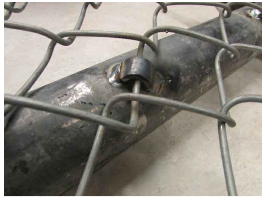
4 CHAIN LINK FENCE FABRIC CURVED GALVANIZED STEEL CLIPS A1.2 SCALE - NTS
