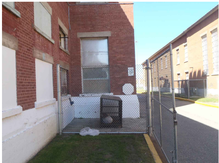
21 FENCE MISSING TOP RAIL
