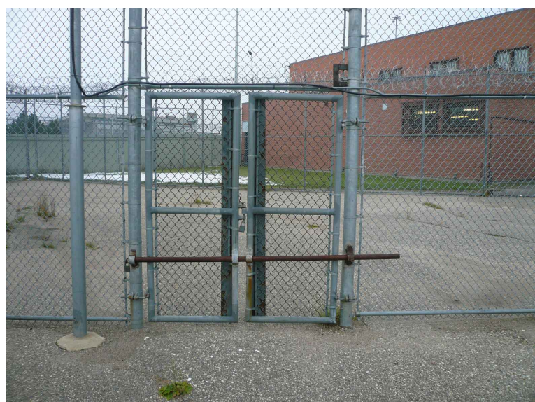
30 SANDBLAST RUST OFF GATE AND PAINT AS NOTED
