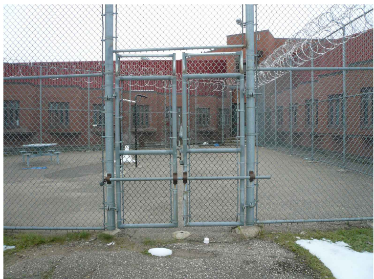
28 SANDBLAST RUST OFF GATE AND PAINT AS NOTED
