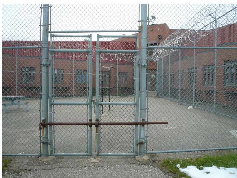
29 SANDBLAST RUST OFF GATE AND PAINT AS NOTED
