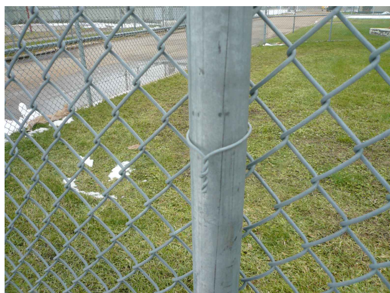
33 CORRECTLY TIED FENCE POST - TIE WIRE IS CORRECTLY TWISTED. BEND TWIST TO POST.
