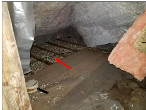
Photo 1. Vermiculite insulation between floor joists in the attic.
