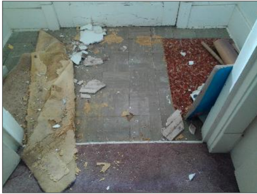
Photo 4. Grey with white streaks vinyl floor tile in the back entrance (Loc. 5).
