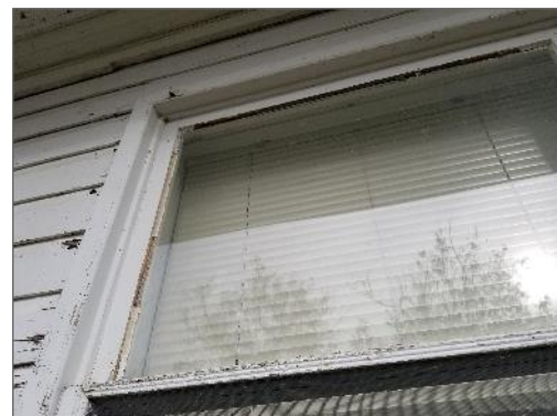
Photo 7. Non-asbestos containing grey caulking around exterior window frames.
